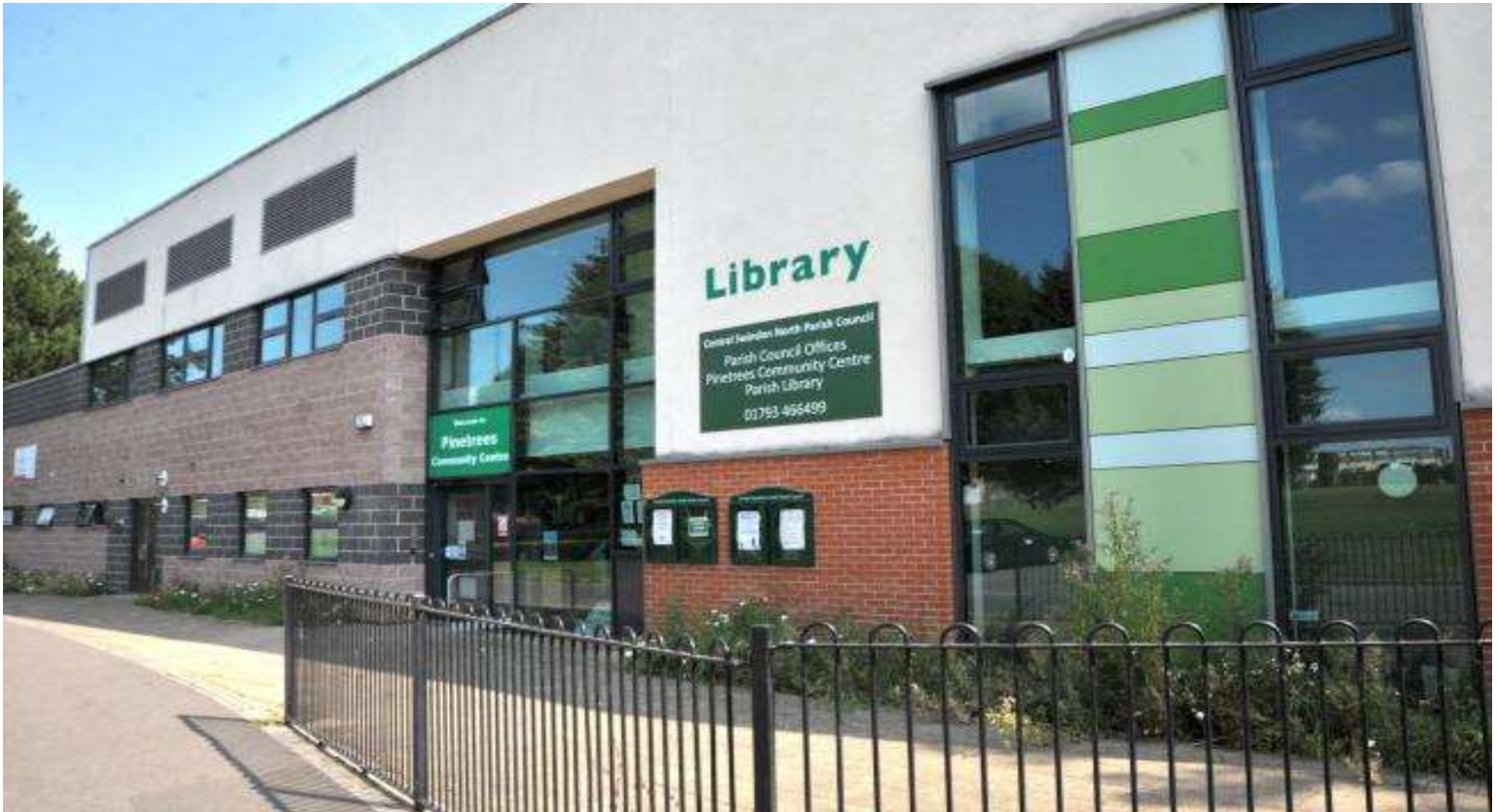
Photo of the Exterior of the Pinetrees Community Centre taken in May 2020.
