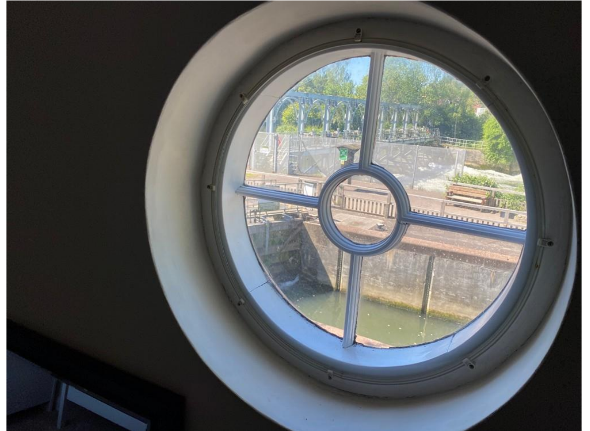
Secondary Glazing to Circular Window
