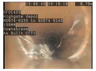
ND074\_0235X\_0e635ae4-788c-4101-af9a-b027c6558970\_20 181018\_194959\_477.jpg, 00:00:03, 0.70 m Roots, fine at joint
