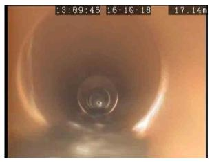
ND074\_0235X\_163291e0-75ac-48ef-95a2-2527c8609293\_20 181018\_195117\_299.jpg, 00:01:05, 17.14 m Fracture, circumferential at joint from 8 o'clock to 10 o'clock
