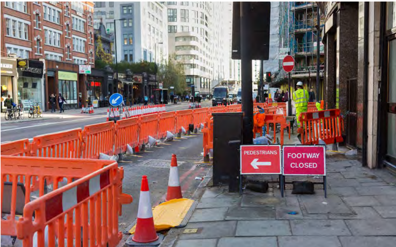
Closed footway with temporary walkway in carriageway
