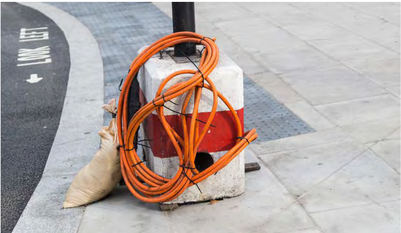
PTS cables should not be easily accessible
