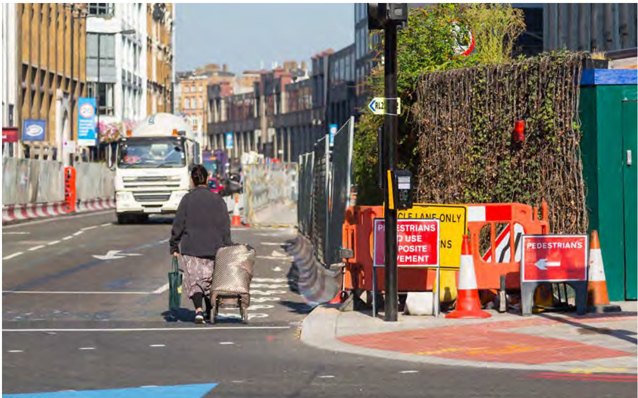
Poor sign usage and clutter
