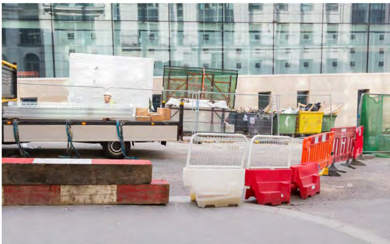
Bad practice: multitude of mixed barrier types, which are not assembled into a continuous barrier
