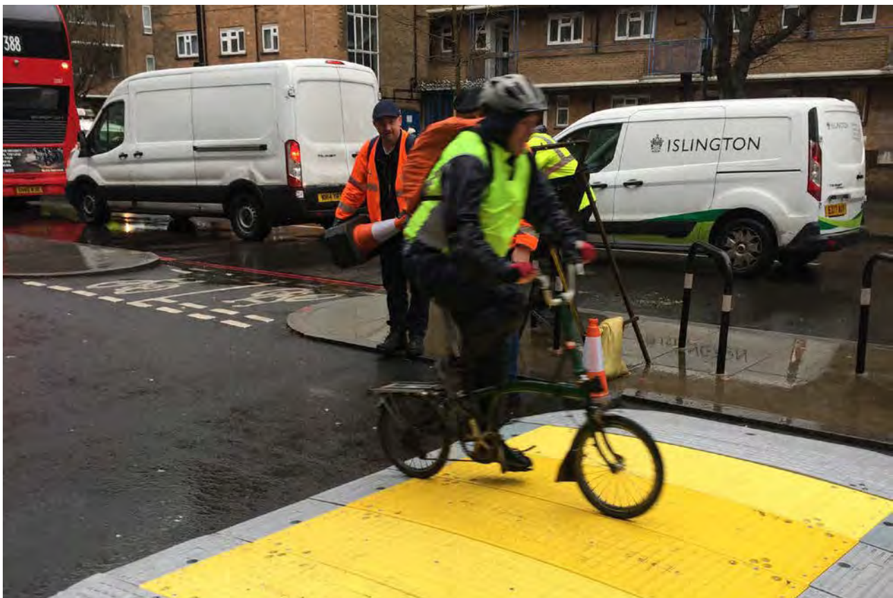
Cycle track road plating system
