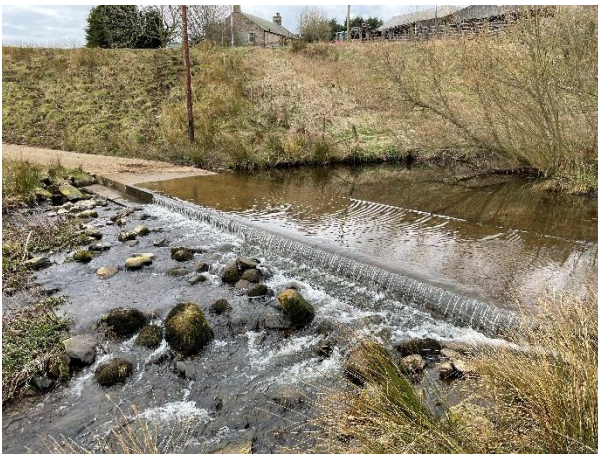
F. Concrete ford structure impounds flow and sediment and limits longitudinal ecological connectivity.
