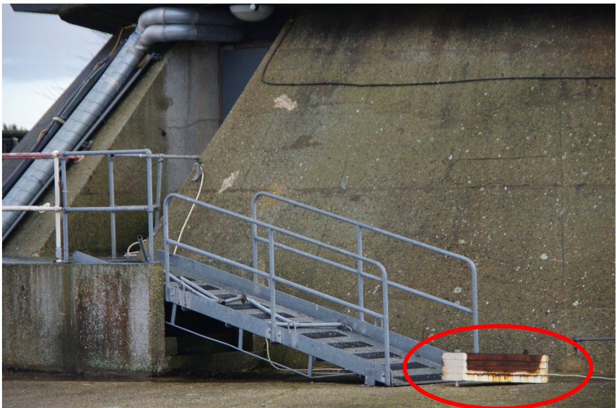
Figure 3. View of fallen counterweight block on apron below 25m antenna.
