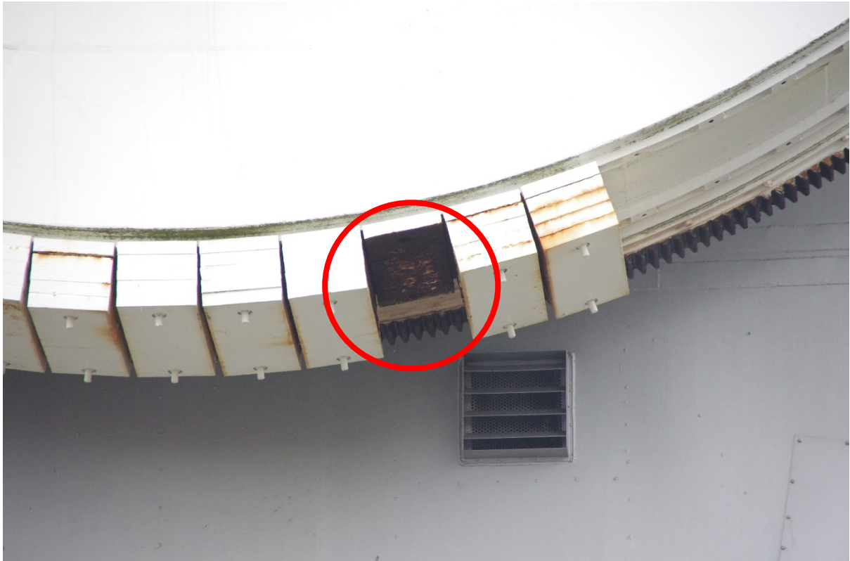
Figure 2. Close up of the missing counterweight block.
