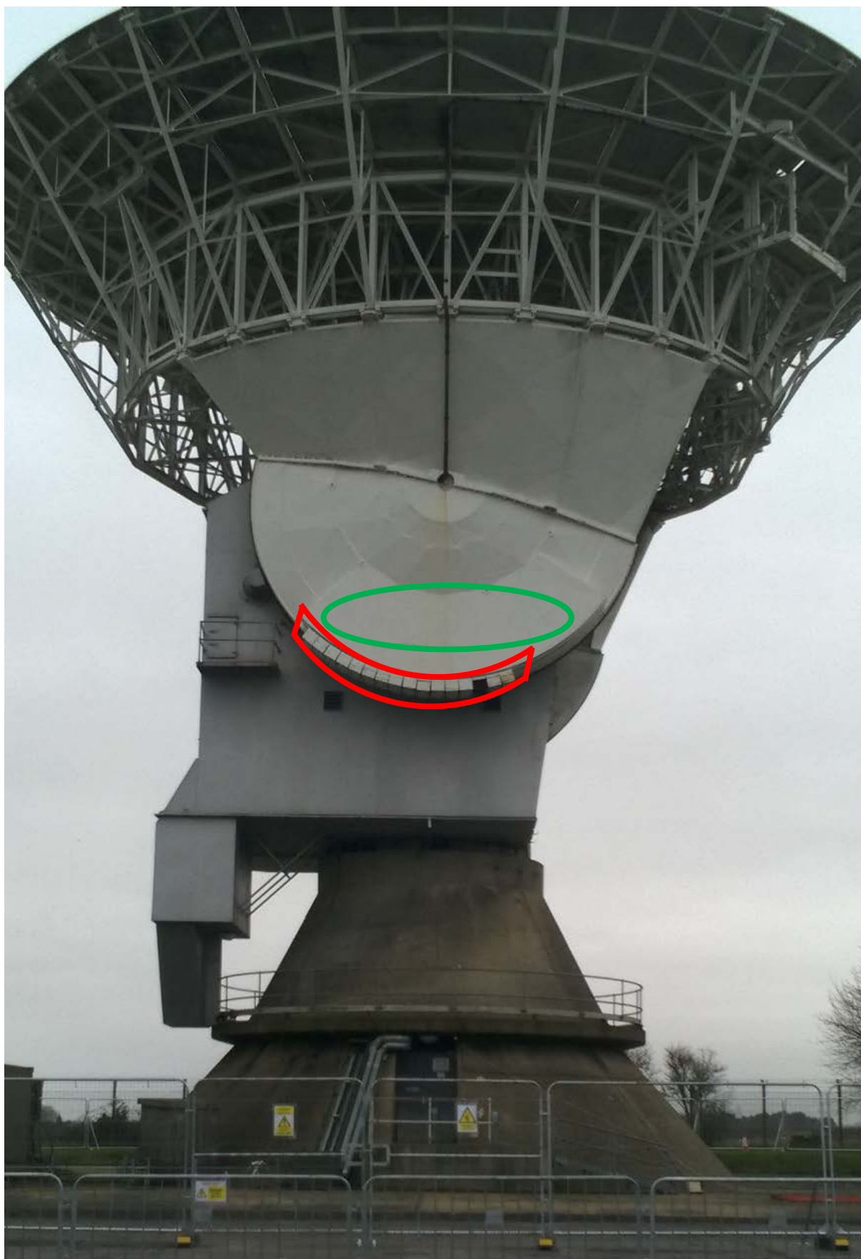
Figure 1. View of Chilbolton Observatory 25m Antenna showing the ballast tank (green) and the counterweight blocks (red).
