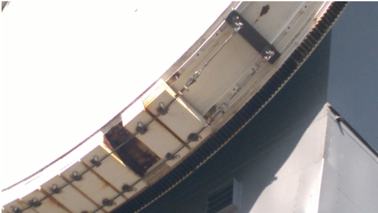
Figure 4. View of the temporary fix to make the situation safe from further block falls.
