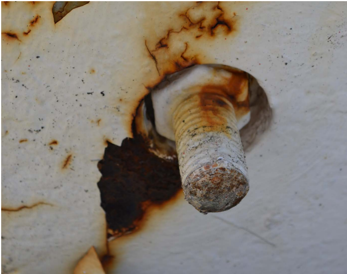
Figure 10. Close-up of stud and nut holding plate.
