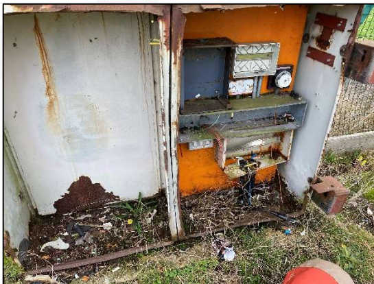
Figure 16 – Damaged electrics
