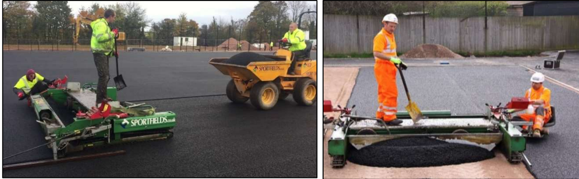
Figure 19 – Example of an insitu laid shock pad
