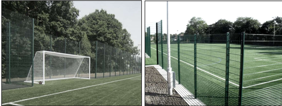
Figure 28 – Example of perimeter ball-stop fencing (rigid mesh ball-stop fencing panel 868 gauge finished RAL6005 Dark Green)
