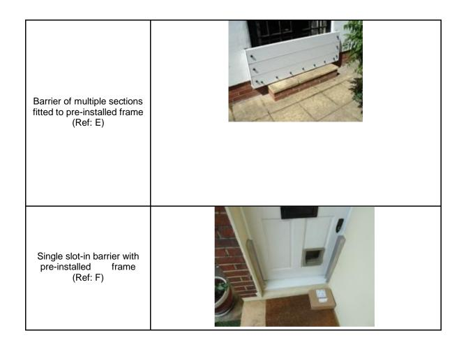
A barrier will include all fixings and all necessary modifications to existing door and surroundings and installation of required permanent fittings and frames, all necessary reinstatement, durable silicone based sealant around the frame, matching the existing and to the required protection height, and around sills to seal all gaps.
