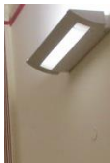
Recessed Wall Mounted Downlight
