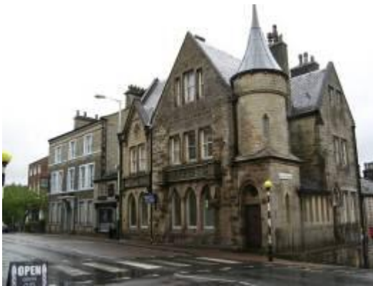
Nos. 18 and 20 Market Street
