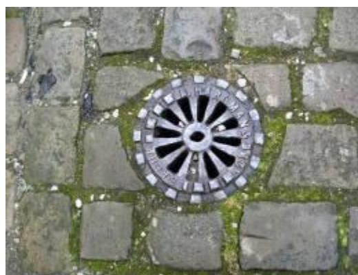
Drain cover in Bank Street
