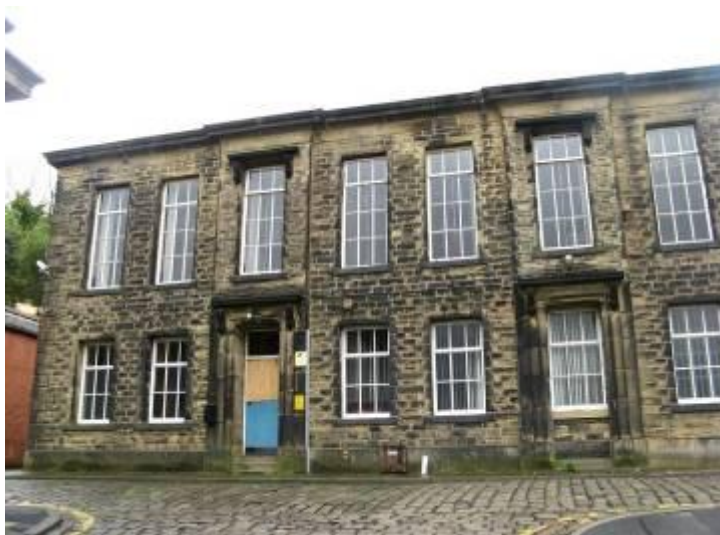
Former Police Station, Bank Street
