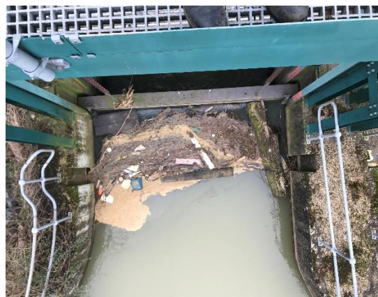
Photo 5 – Middle sluice light position
