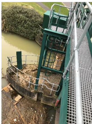
Photo 4 – Vertical access ladder
