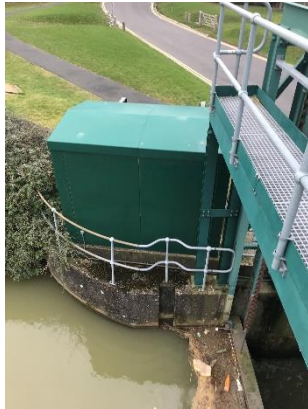
Photo 6 – High level walkway
