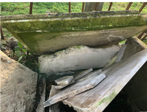
Detail of fractured south base panel of monument
