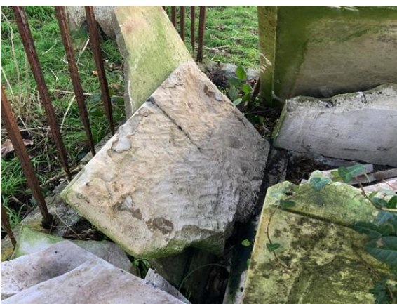
Detail of fractured east base panel of monument
