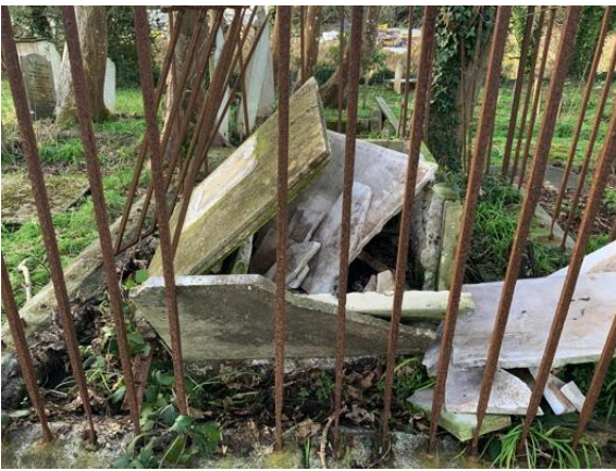
Detail of fragmented marble panels within and outside monument base
