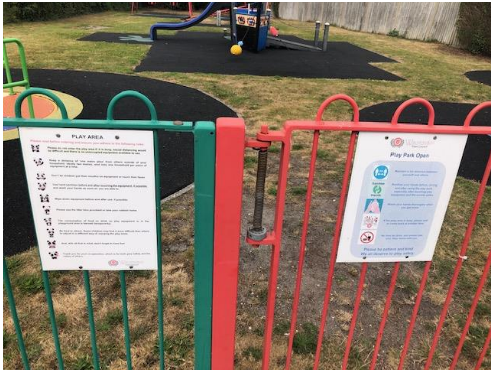
Pedestrian Gate to be re-furbished with 2 new coats of paint, closing mechanism and springs to be checked. New sign to be installed onto steel post.
