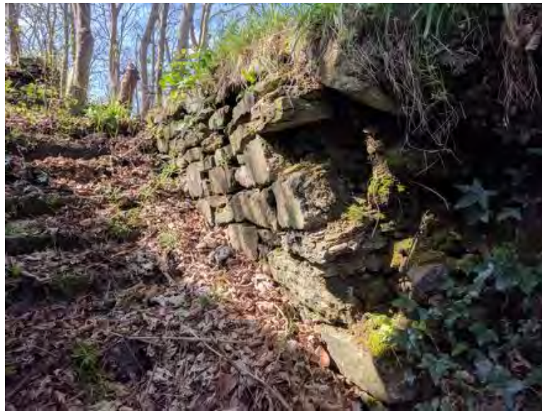
Figure 51 Collapsed inner face of western stairwell wall
