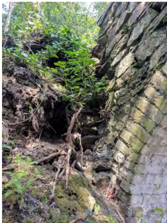
Figure 48 Detail view of rear of Arch intersection with earth bank and collapsed western stairwell wall
