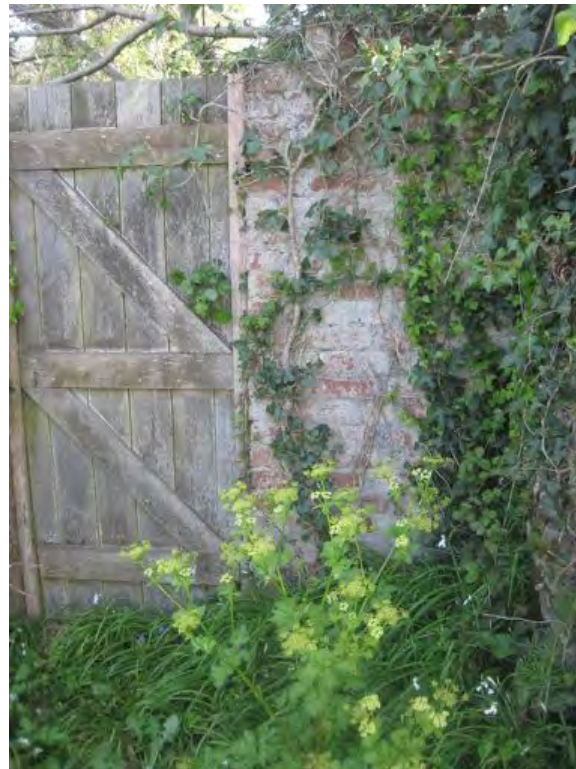
Figure 5 Brickwork wall to RHS of gateway, some missing coping bricks to wall head
