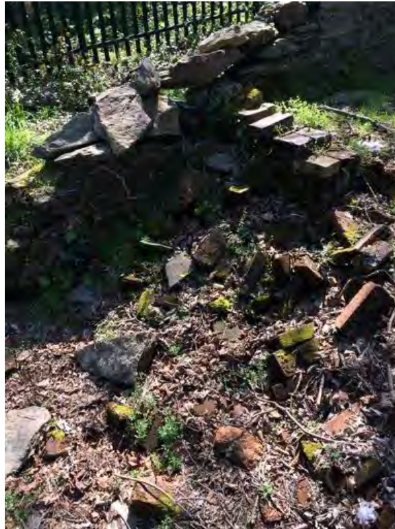
Figure 58 Detail view of collapsed brickwork within footprint of building
