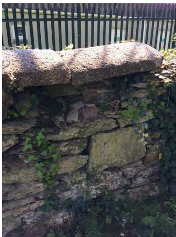
Figure 31 (8m) Detail of granite copings and deep pointing voids to stonework
