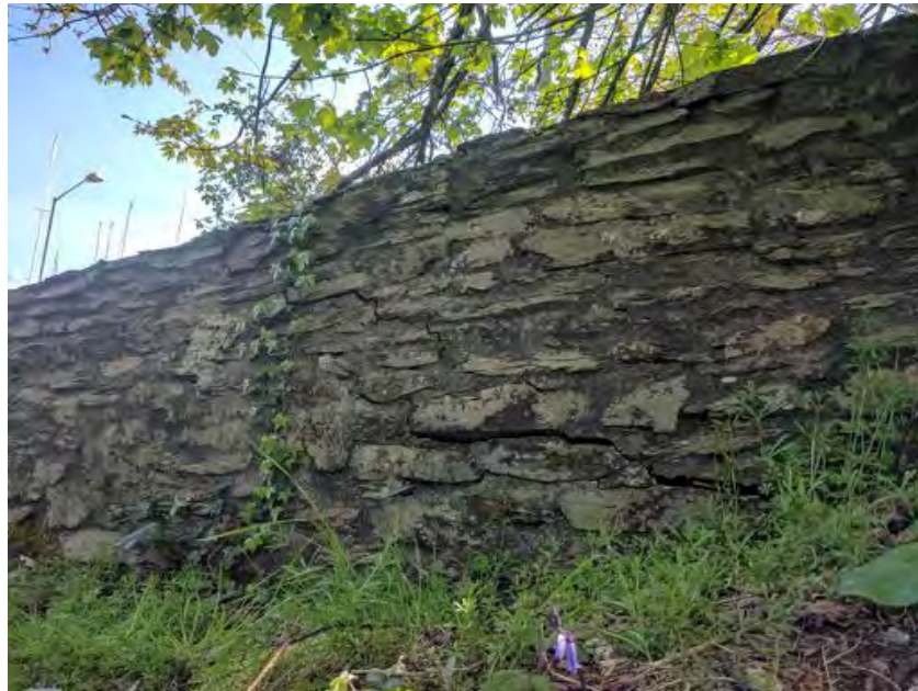
Figure 26 (approx 1m-4m) note the minor cracking to concrete coping and significant crack to centre of photograph
