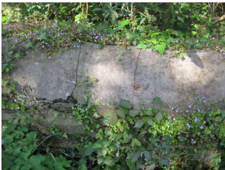
Figure 4 Detail of concrete coping to B1. Note cracking and damage (this is one of the best preserved sections)
