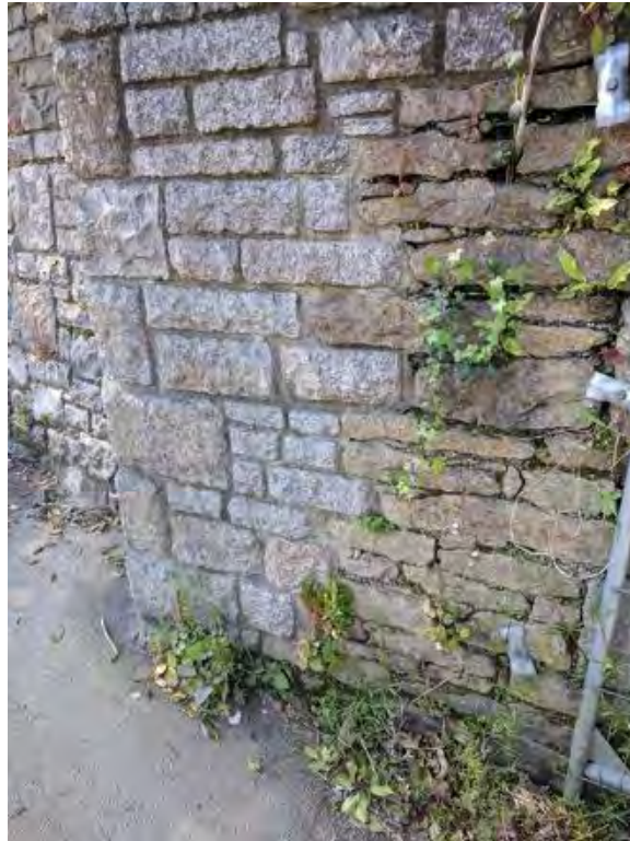
Figure 47 Detail of how contemporary retaining wall was constructed to tie into existing masonry
