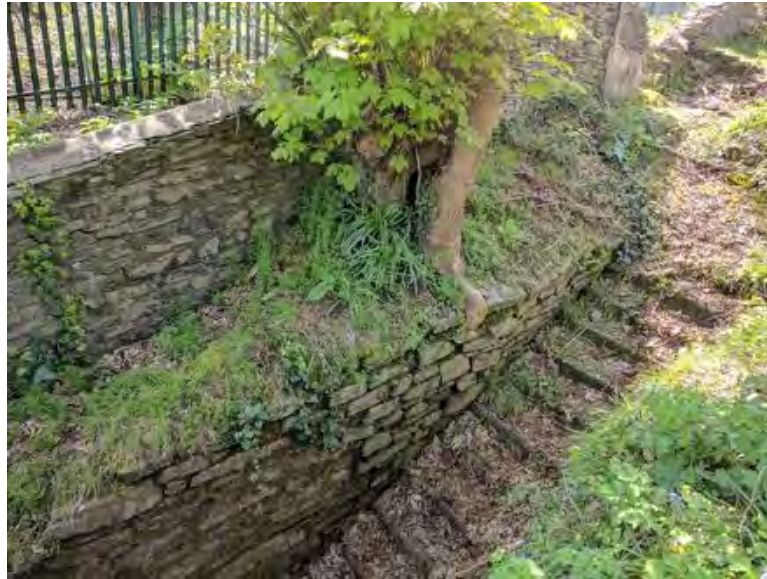
Figure 55 General view of eastern stairwell wall showing CT20 growing from wall head
