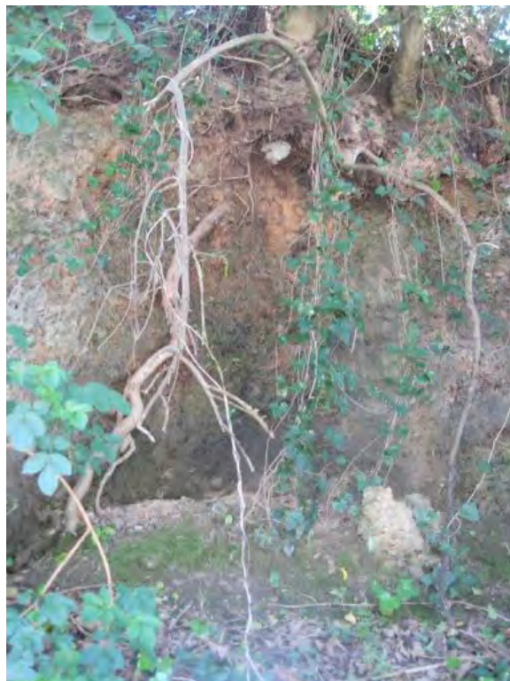
Figure 24 Detail of bank from below - note areas of substantial collapse
