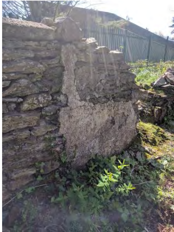
Figure 32 Detail of render remains at approx. 8m-9m length
