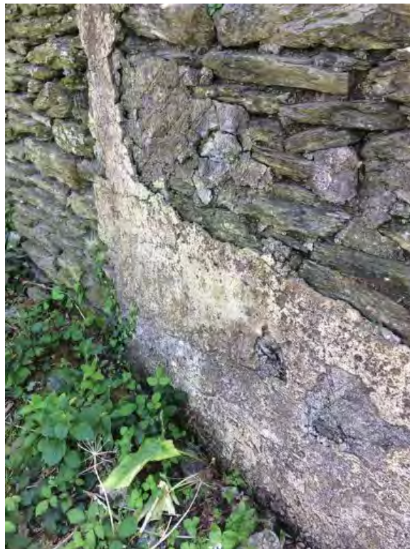
Figure 59 Detail of render/plaster remains to boundary wall
