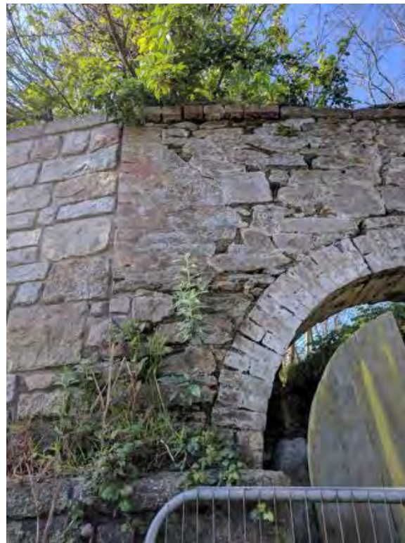
Figure 46 Junction of existing arch with contemporary stone retaining wall
