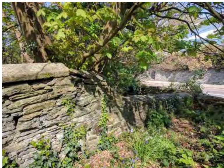
Figure 29 Detail of step change in wall at approx. 4m-5m.
