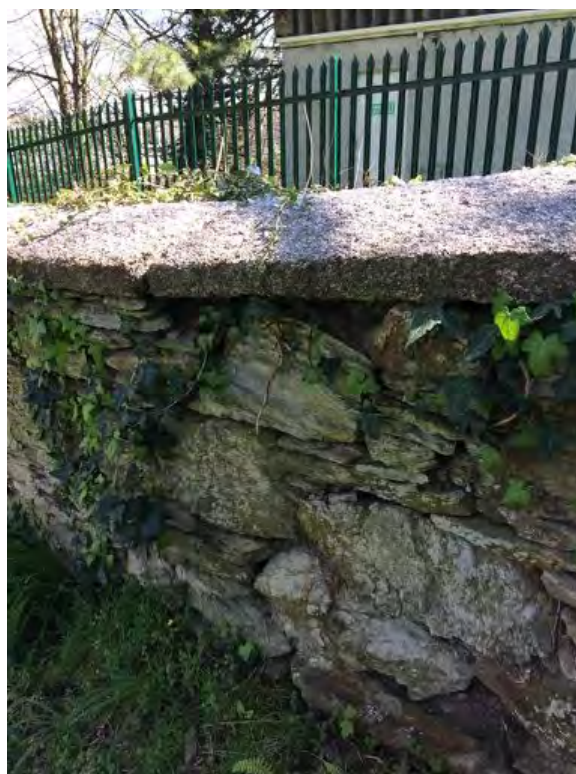
Figure 30 (4-8m) Section of B6 in good condition, coping stones need some re-bedding and stonework repointing.
