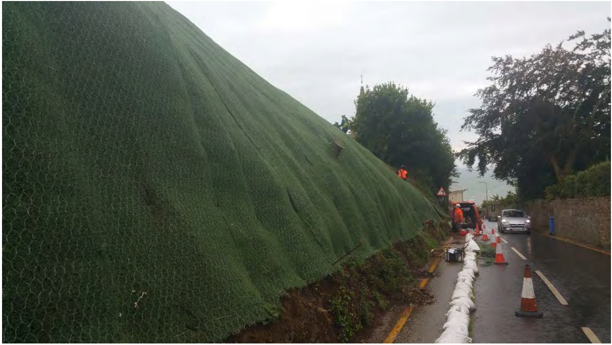
Figure A: MACMAC-R (Green) being installed on a similar site.
