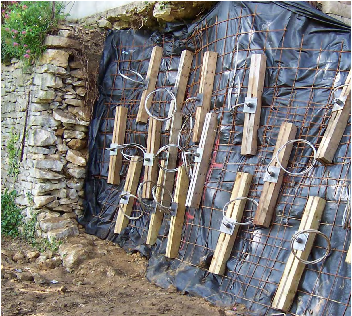
Figure B: Potential alternative method of stabilising material behind west stairwell wall.
