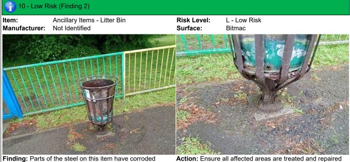
excessively and the metal has perforated in places
