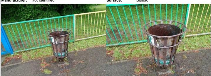
Finding: There is some evidence of fire damage to the item Action: Monitor for any further deterioration and repair as required
