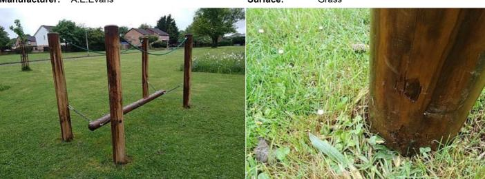
Finding: There is some strimmer / machinery damage apparent on the posts, this can penetrate the preservative applied to the timber and accelerate the rotting process
