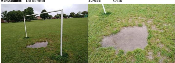
**Finding:** The surface has eroded in some areas and may be **Action:** Reinstate the surface slippery in wet conditions
