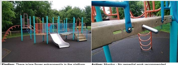
Finding: There is/are finger entrapment/s in the platform and the item fails to meet the requirements of BS EN 1176 Part 1 4.2.7.6 Entrapment of fingers
