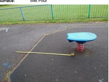
**Finding:** The surfacing dimensions are short and do not meet with the requirements of the current applicable standard
