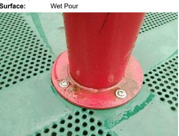
Finding: The paintwork on this item has been damaged or Action: Treat affected areas and repaint worn exposing the metal underneath which is rusting / corroding
