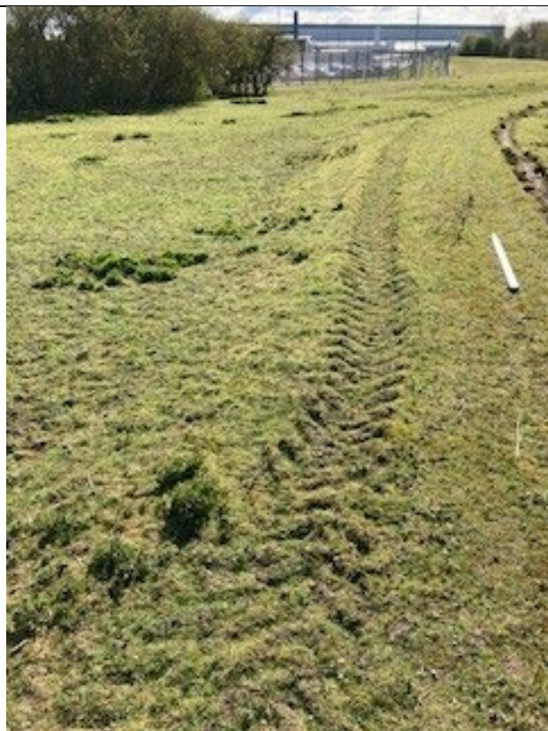
Damage from tracked plant on crest
