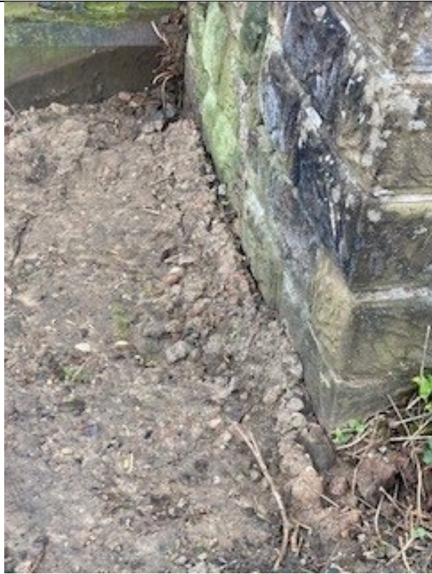
Loose fill from trial pit
