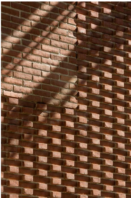
Projecting header brick patterns
