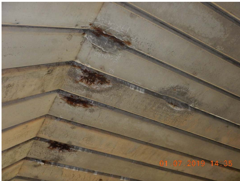
1.2: Typical areas of spalling and corrosion to the reinforcement within the portal beams.
