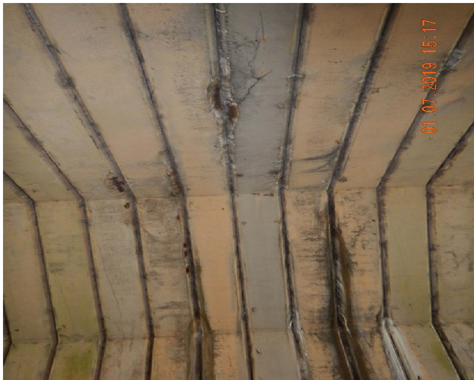
2.2: Typical areas of spalling and corrosion to the reinforcement within the portal beams.
