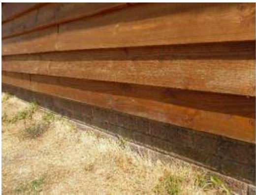
Red Brick Plinth and Douglas Fir Feather edge boarding, 200mm x 12-25mm.
