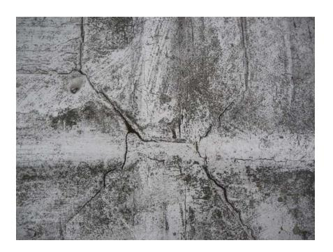
Surface cracks/crazing in the roof felt and coating
