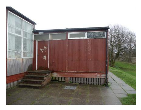
Typical elevation. The floor is rotten by the door
