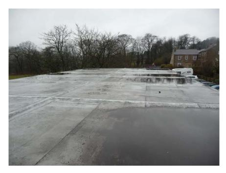
Roof over the hall. Ponding due to inadequate fall
