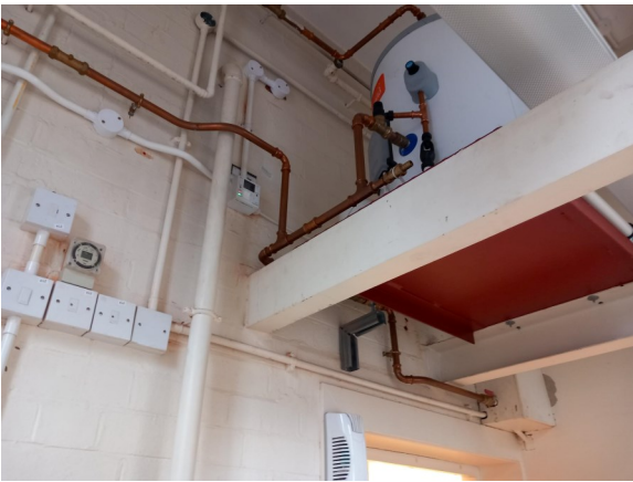
High Level Hot Water Heater above DDA Toilet
