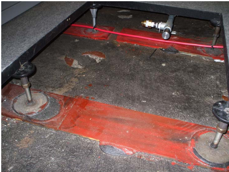
■ Figure 5: Raised floor and spreader plate arrangement
