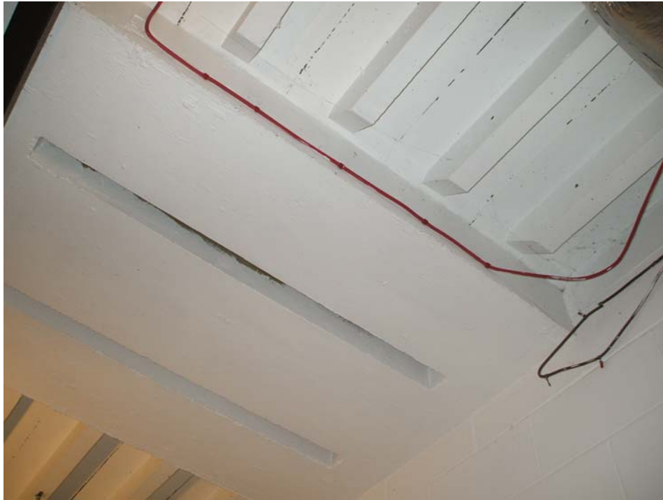
■ Figure 4: "T" PC planks and main beam
