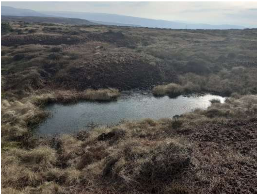
Figure 4: Example of Gully block pool - peat dam on left. Dams can be stone, timber, plastic, heather bale or coir log.
