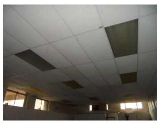
Lower Ground (East Wing) Floor: Area: Room LG85 Location: To Ceiling Above False Ceiling **Description:** Paper-Lined Tiles & Bitumen Adhesive Extent: m2 Accessibility: 2. Above a suspended ceiling, floor or wall void, service or plant area, loft or cellar
