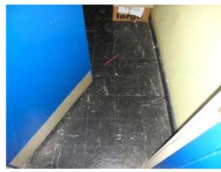
Floor: Second Floor (East Wing) Internal Area: Room 276 Location: To Floor **Description:** Black Vinyl Tiles & Bitumen Adhesive Extent: m2 Accessibility: 4. Easily accessed, below head height
