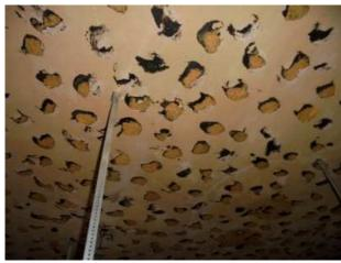
Floor: Second Floor (East Wing) Internal Area: Room 256 Location: To Ceiling Above False Ceiling **Description:** Paper-Lined Tiles & Bitumen Adhesive Extent: m2 Accessibility: 2. Above a suspended ceiling, floor or wall void, service or plant area, loft or cellar
