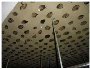
Floor: First Floor (West Wing) Internal Area: Room 108 Location: To Ceiling Above False Ceiling Description: Paper-Lined Tiles & Bitumen Adhesive Extent: m2 Accessibility: 2. Above a suspended ceiling, floor or wall void, service or plant area, loft or cellar
