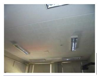
Second Floor (East Wing) Internal Floor: Area: Room 254 Location: To Ceiling **Description:** Paper-Lined Tiles & Bitumen Adhesive Extent: Accessibility: 3. Exposed overall, but above head height
