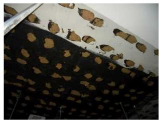
Floor: First Floor (West Wing) Internal Area: Room 106 Location: To Ceiling Above False Ceiling **Description:** Paper-Lined Tiles & Bitumen Adhesive Extent: m2 Accessibility: 2. Above a suspended ceiling, floor or wall void, service or plant area, loft or cellar
