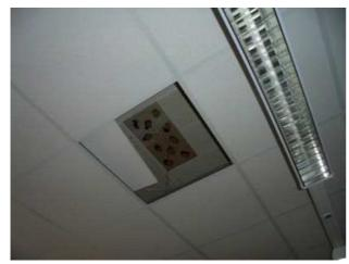
Ground Floor (East Wing) Internal Floor: Area: Room G56 Location: To Ceiling Above False Ceiling **Description:** Paper-Lined Tiles & Bitumen Adhesive Extent: Accessibility: 2. Above a suspended ceiling, floor or wall void, service
