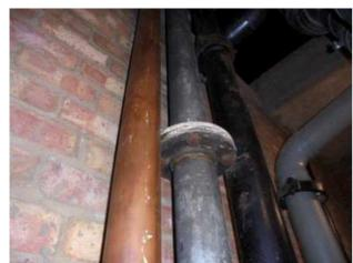
Floor: Fourth Floor (West Wing) Area: Male WC Location: Within Riser to Left of Male WC Description: Gasket to Pipe Join Extent: Extensive Accessibility: 2. Above a suspended ceiling, floor or wall void, service
