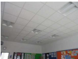
Floor: First Floor (East Wing) Internal Area: Room 167 Location: To Ceiling Above False Ceiling **Description:** Paper-Lined Tiles & Bitumen Adhesive Extent: m2 Accessibility: 2. Above a suspended ceiling, floor or wall void, service or plant area, loft or cellar
