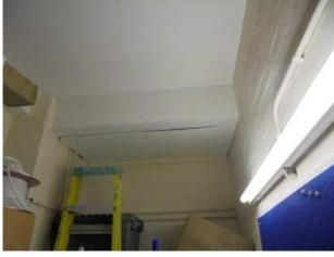
Floor: Ground Floor (East Wing) Internal Area: Room G66 Location: To Ceiling **Description:** Paper-Lined Tiles & Bitumen Adhesive m2 Extent: Accessibility: 3. Exposed overall, but above head height
