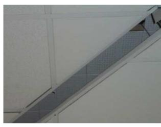
Floor: Ground Floor (East Wing) Internal Area: Room G52 & G53 Location: To Ceiling **Description:** Paper-Lined Tiles & Bitumen Adhesive m2 Extent: Accessibility: 3. Exposed overall, but above head height
