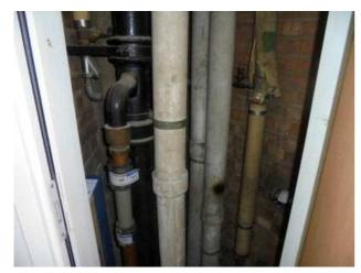
Fourth Floor (West Wing) Internal Floor: Area: Male WC Location: Within Riser **Description:** Cement Flue Pipes Extent:
