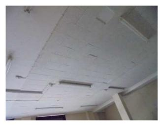
First Floor (East Wing) Floor: Internal Area: Room 162 Location: To Ceiling **Description:** Paper-Lined Tiles & Bitumen Adhesive m2 Extent: Accessibility: 3. Exposed overall, but above head height
