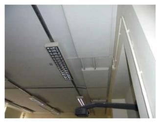
Second Floor (West Wing) Floor: Internal Area: Room 204 & 205 Location: To Ceiling **Description:** Thermal Insulation Within Panels Extent: Qty Accessibility: 1. Reachable only with hands (via a inspection hatch)
