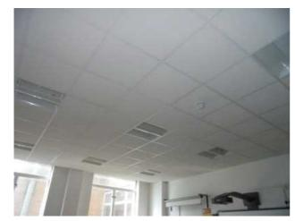
Second Floor (East Wing) Internal Floor: Area: Room 270 Location: To Ceiling Above False Ceiling **Description:** Paper-Lined Tiles & Bitumen Adhesive Extent:
