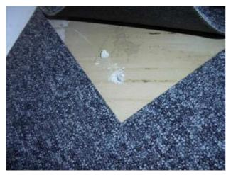
Floor: Fourth Floor (West Wing) Internal Area: Room 401 Location: Below Floor Screed Description: Bitumen Adhesive m2 Extent: 4. Easily accessed, below head height Accessibility:
