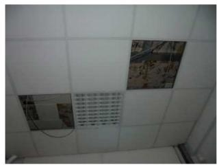
Floor: Ground Floor (East Wing) Internal Area: Room G54A Location: To Ceiling Above False Ceiling **Description:** Paper-Lined Tiles & Bitumen Adhesive Extent: m2 Accessibility: 2. Above a suspended ceiling, floor or wall void, service or plant area, loft or cellar
