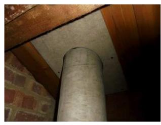
Floor: Third Floor (West Wing) Internal Area: South Large Loft Space Location: To Underside of Roof **Description:** Cement Flue Exit Plate Extent: m2 **Accessibility:** 2. Above a suspended ceiling, floor or wall void, service
