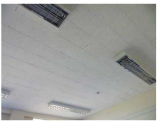
Second Floor (East Wing) Internal Room 253 Location: To Ceiling **Description:** Paper-Lined Tiles & Bitumen Adhesive m2 Accessibility: 3. Exposed overall, but above head height
