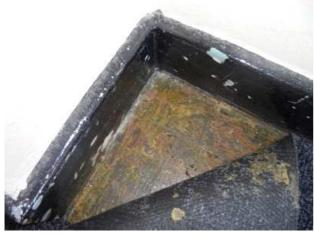
Floor: Second Floor (East Wing) Internal Area: Room 292 Location: To Floor **Description:** Floor Tiles & Bitumen Adhesive m2 Extent: Accessibility: 4. Easily accessed, below head height
