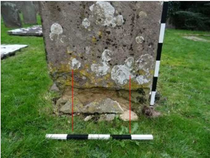
Suggested location for stainless steel supports.
