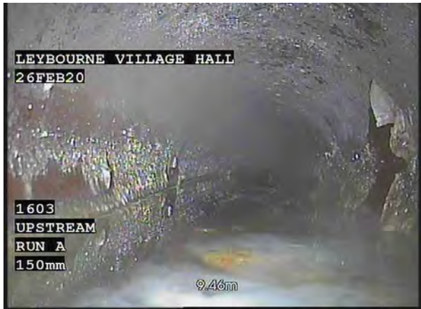
1, 00:00:45, 9.46 m Water level, 60% of the vertical dimension, Standing water - irregular gradient or backfall
