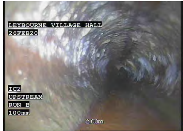
2, 00:00:42, 2.00 m Attached deposits, grease from 08 o'clock to 04 o'clock, 10% cross-sectional area loss, start
