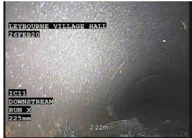
2, 00:00:44, 2.22 m Settled deposits, fine, 45% cross-sectional area loss, start
