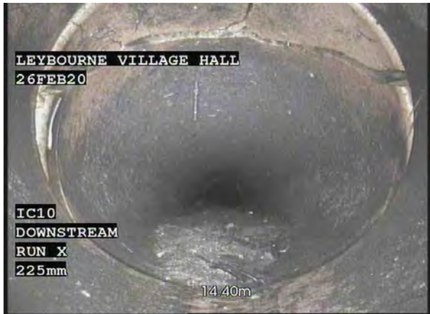
1, 00:01:06, 14.40 m Fracture, multiple at joint from 12 o'clock to 12 o'clock
