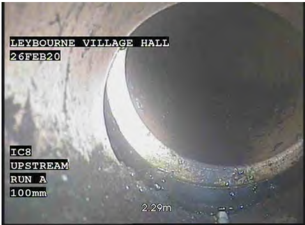
1, 00:00:19, 2.29 m Joint displaced, large
