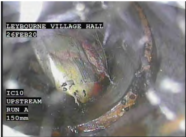
1, 00:01:48, 7.13 m Settled deposits, coarse, 80% cross-sectional area loss
