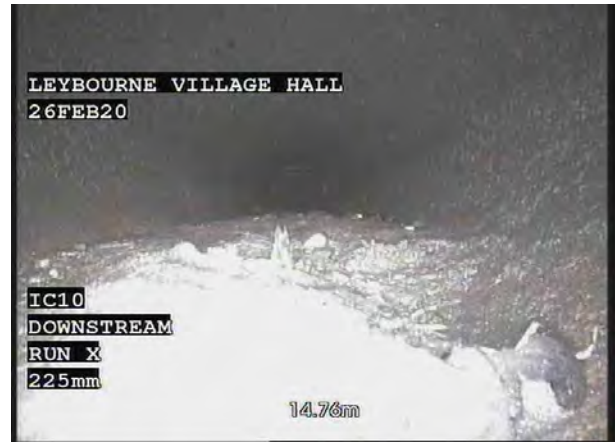
2, 00:01:19, 14.76 m Settled deposits, fine, 15% cross-sectional area loss, start
