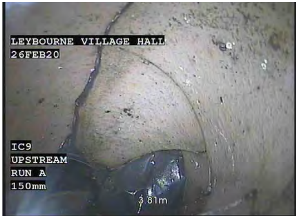
1, 00:01:24, 3.81 m Fracture, multiple from 12 o'clock to 12 o'clock
