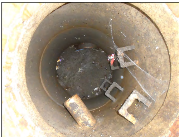
IC12 CATCHPIT SILTED
