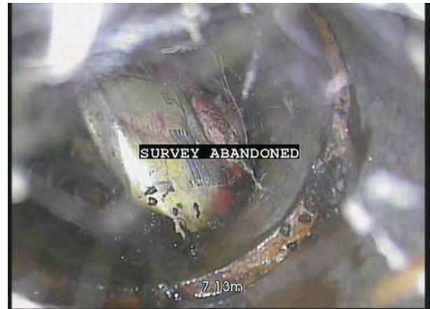
2, 00:01:57, 7.13 m Survey abandoned, Unable to pass
