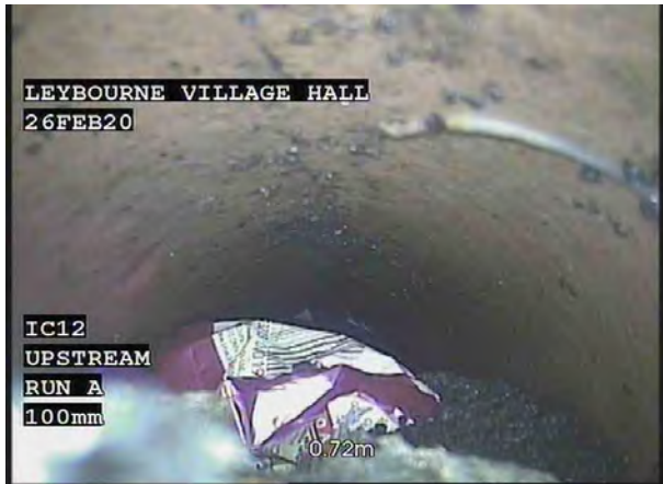
1, 00:00:18, 0.72 m Settled deposits, coarse, 70% cross-sectional area loss
