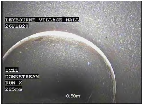
1, 00:00:12, 0.50 m Settled deposits, fine, 25% cross-sectional area loss, start
