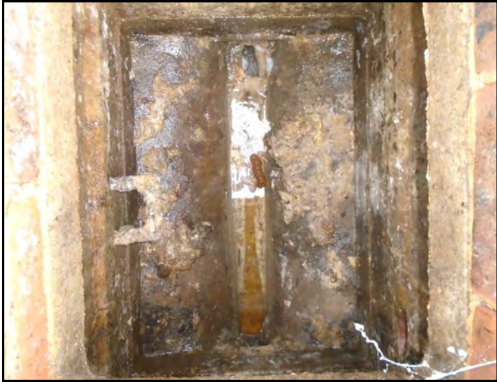
IC2 BACKFALL IN CHAMBER
