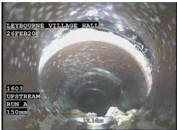
3, 00:01:31, 12.14 m Joint displaced, large
