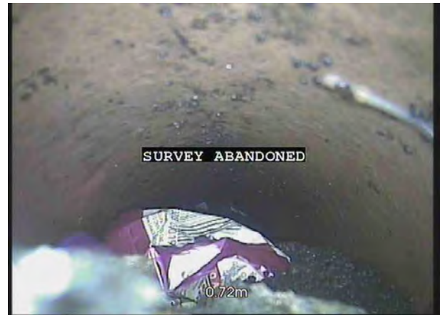
2, 00:00:24, 0.72 m Survey abandoned, Unable to pass
