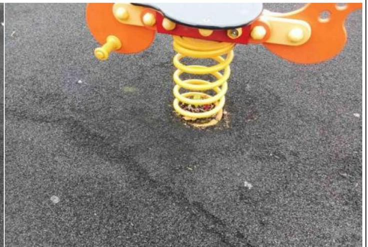
**Finding:** The surface has subsided in some areas **Action:** Monitor for any further deterioration and repair as required
