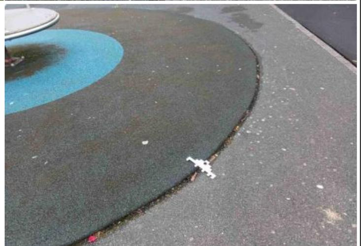
**Finding:** There are significant gaps (over 30mm) between the surface and the edging or between the joints in the surface; these are large enough for a small foot to enter
