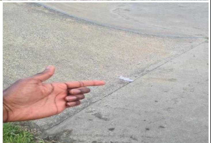
**Finding:** Joints between the riding / rolling surfaces shall not be greater than 5mm in contravention of the requirements of BS EN 14974 – 6.2.4
