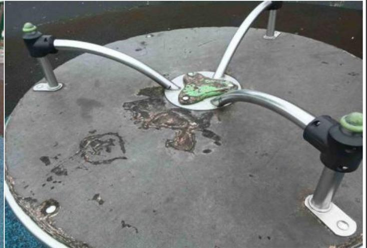
**Finding:** The plywood has delaminated in some places
