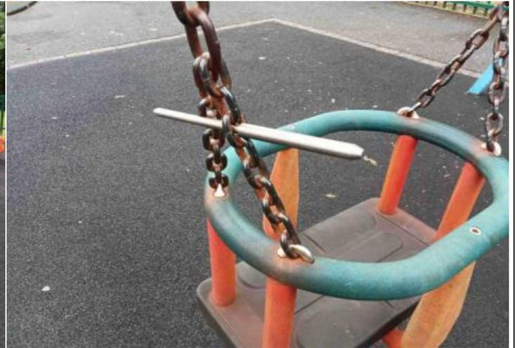
**Finding:** The chain openings are in excess of the 8.6mm as recommended by BS EN 1176 **Action:** Monitor - No remedial work recommended
