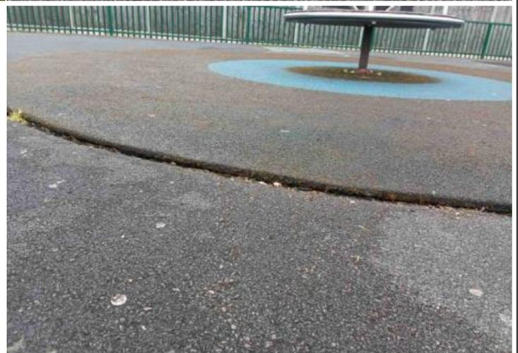
**Finding:** The surface is lifting at the edges and creating trip points **Action:** Repair perimeter of surfacing to remove trip points
