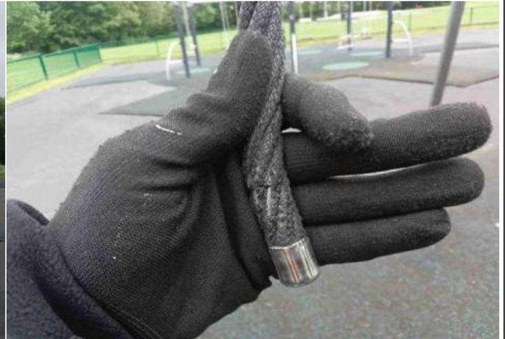
**Finding:** The ropes/nets are worn/damaged in places
