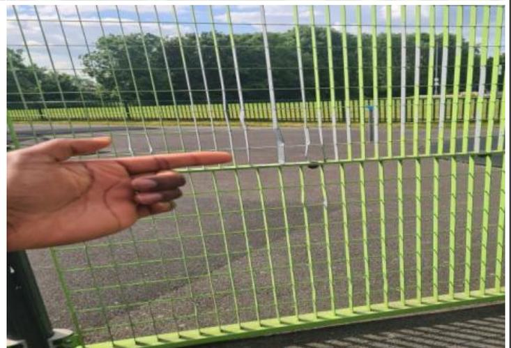
**Finding:** The weld(s) on this item have failed leaving sharp edges
