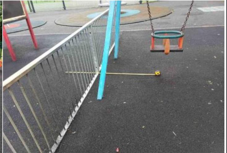
**Finding:** BS EN 1176 Part 2: Annex A makes a recommendation that fences or enclosures should be upto 1.50m from the edges of the swing seat to the sides, and subject to risk assessment, from the edge of the impact area. This is however, a low risk finding and no remedial action is recommended.
