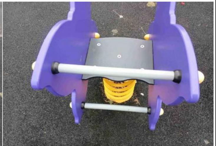
**Finding:** The Handgrips/Footrests rotate and may cause an unexpected movement for the user
