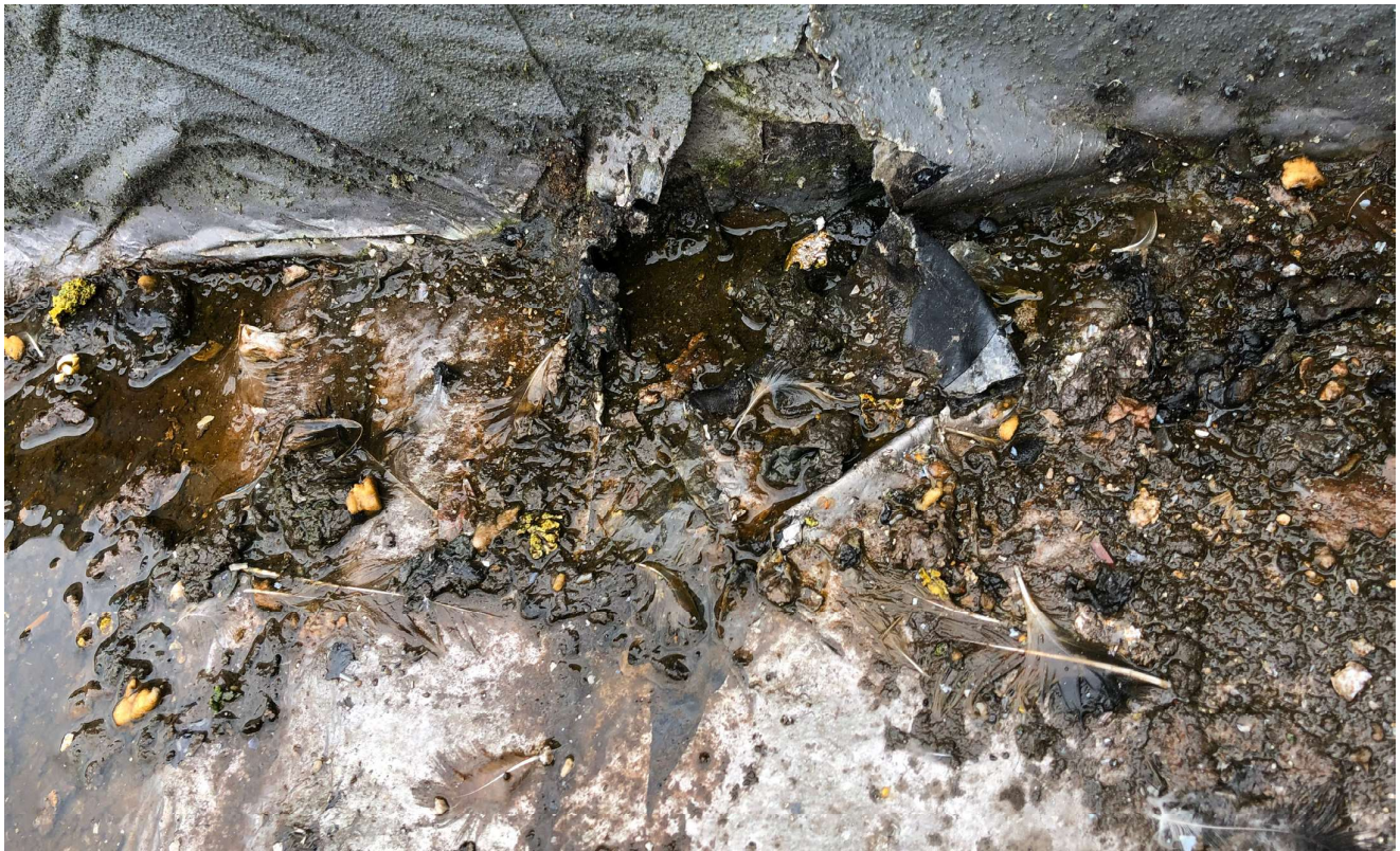
3.4.1 – failed membrane at most joint locations
