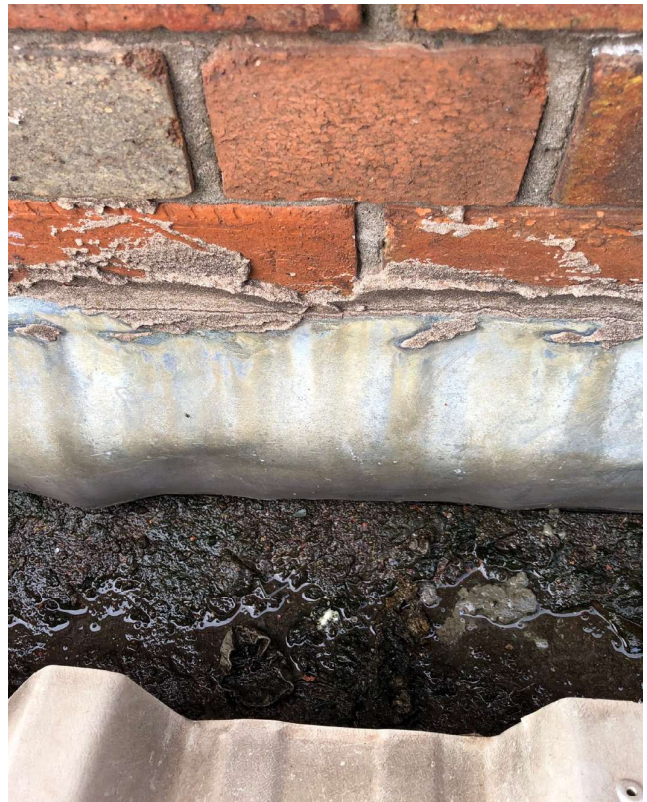
4.4.1 – thick sludge in gutters
