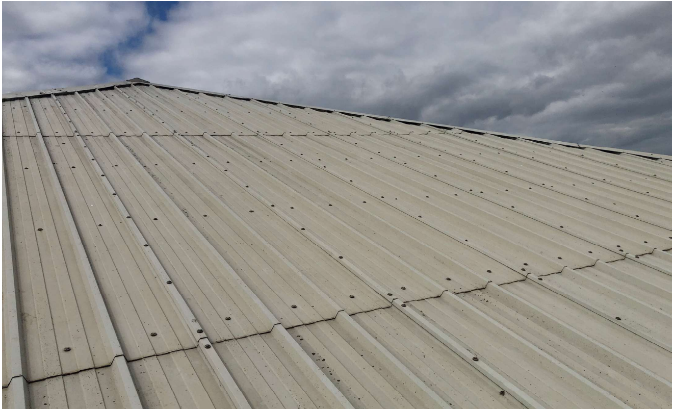
3.2.1 – roof sheets in good condition (Roof A)
