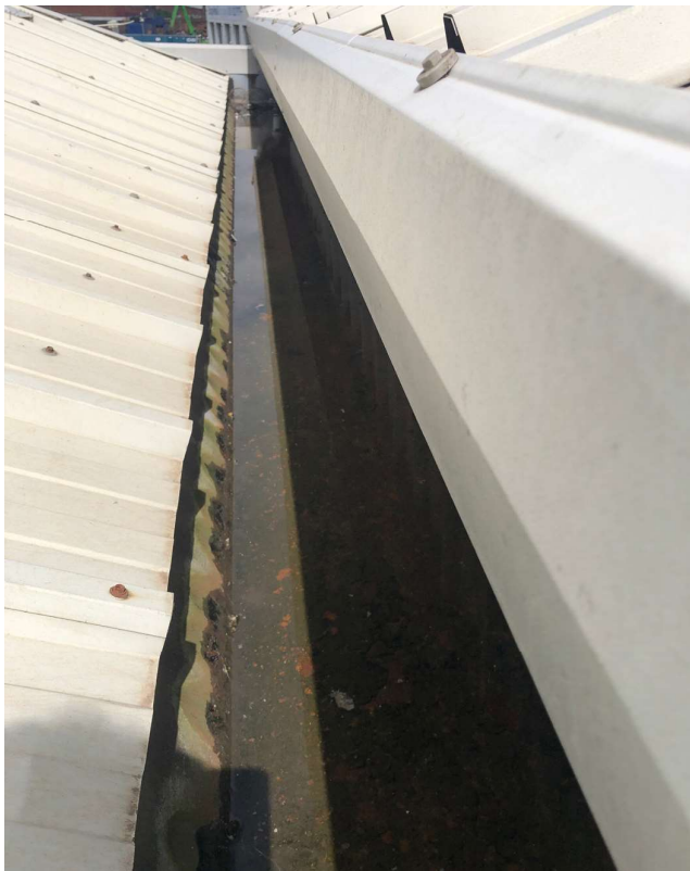
3.4.2 – water ponding which made it difficult to inspect the gutter
