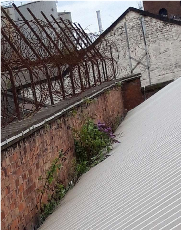
4.3.1 – vegetation needs to be removed from masonry parapet and copings
