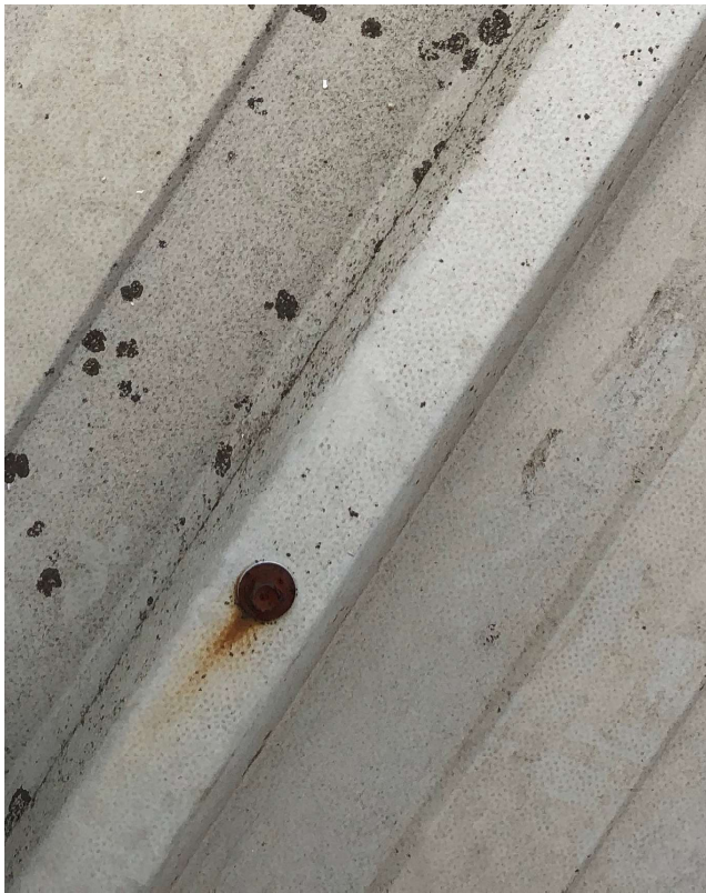
3.2.4 – rusty fixings due to waterproof caps removed (roof sheets)
