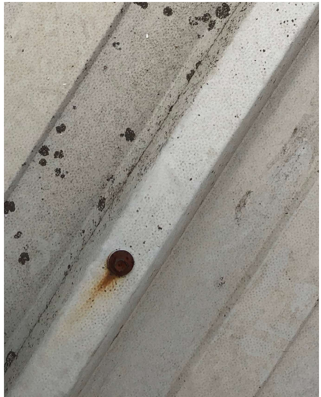
4.2.3 - rusty fixings due to waterproof caps removed (roof sheets)
