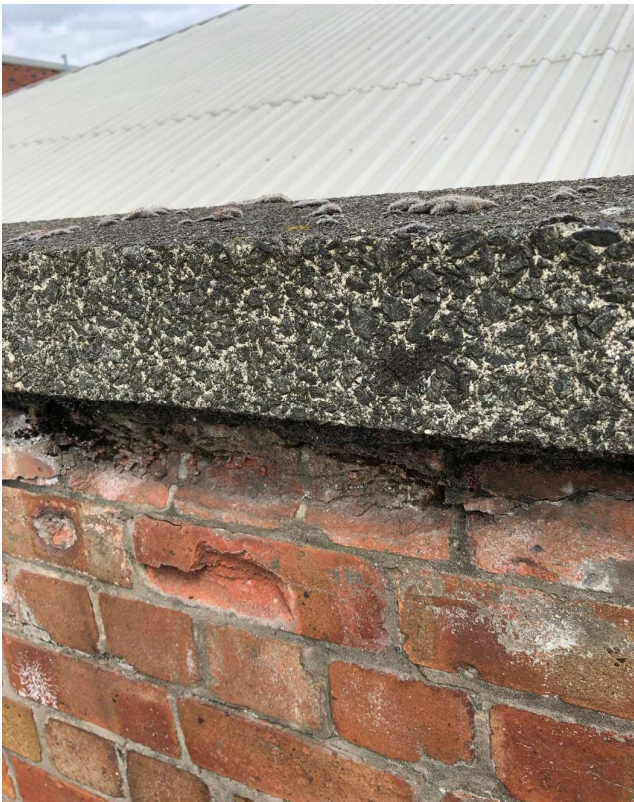
4.3.3 – Spalling of masonry
