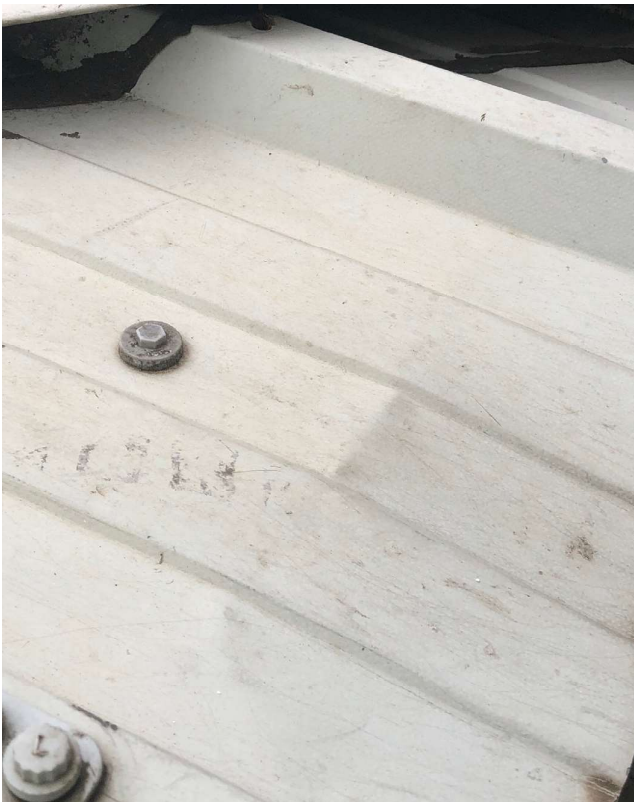
3.6.3 — damaged or depressed flashings
