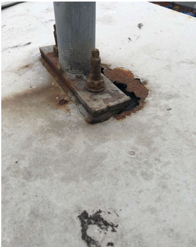
3.3.2 – parapet has corroded due to inappropriate fixings
