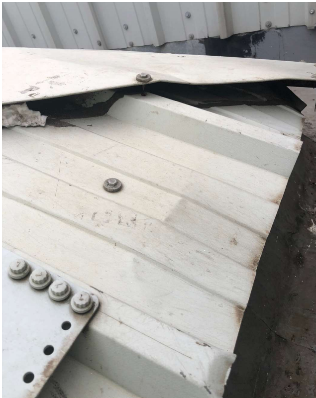
3.2.2 – depressed sheet edges due to being stood on
