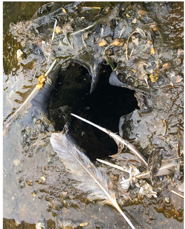
3.5.1 – rainwater outlet in poor condition, with missing leafguard
