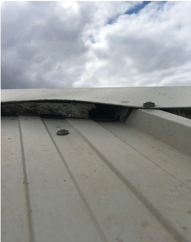
3.6.1 — Missing foam fillers at ridge lines
