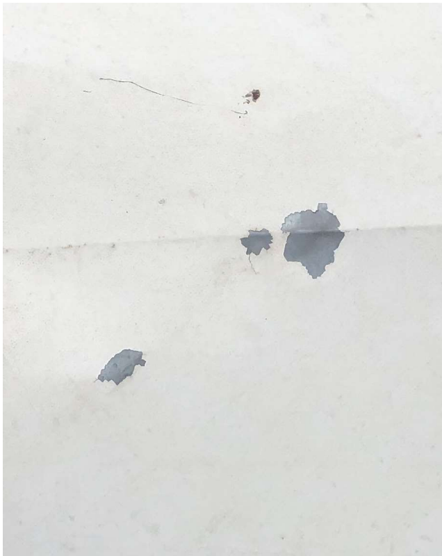
4.2.2 - protective coating removed and bare metal exposed (roof sheets)
