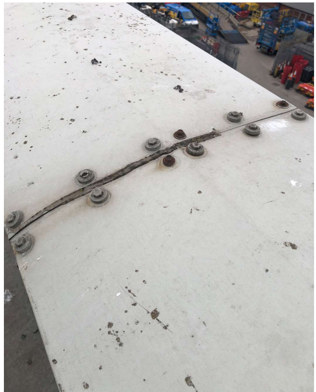
3.3.3 – earlier remedial works in an attempt to seal the gaps (parapet joints)
