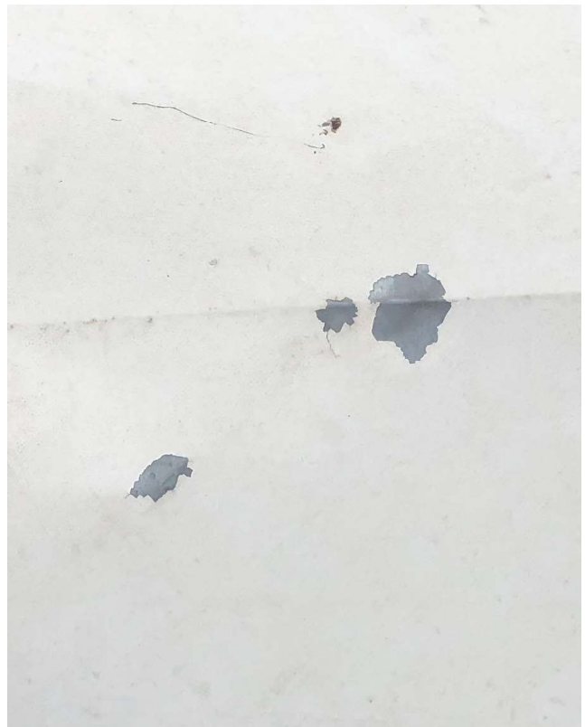
3.3.1 – protective coating removed and bare metal exposed (parapets and copings)
