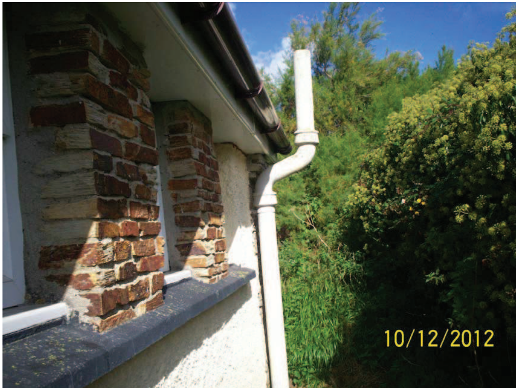
Photo 1: Showing asbestos soil vent pipe
