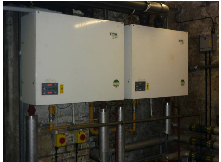
SCC - Gas fired boilers_1.0
