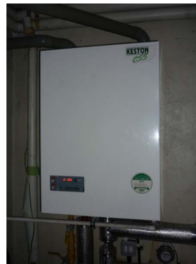
Bothy Building - Gas fired Boiler_1.0
