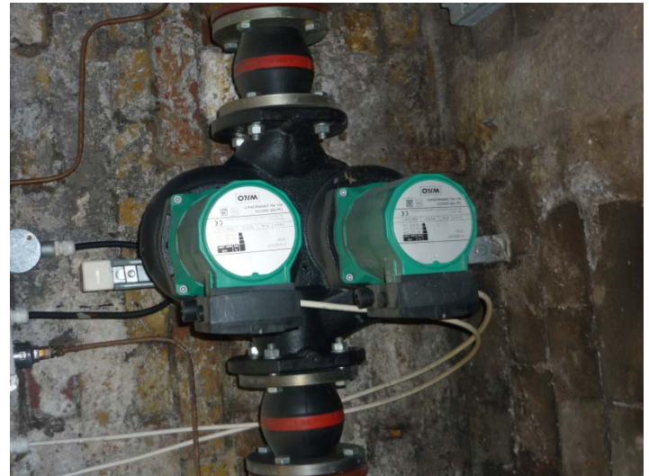
SCC - Main heating circulation pumps_1.0
