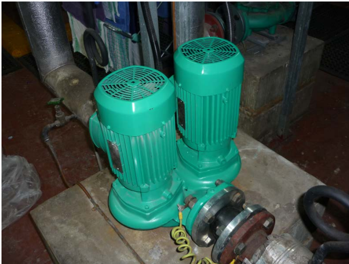
South Hall Boiler room - Basement heating pump set_1.0
