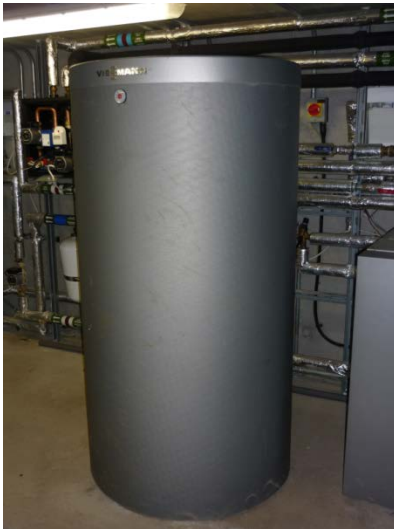
The Pavillion - Hot Water Storage calorfier_1.0
