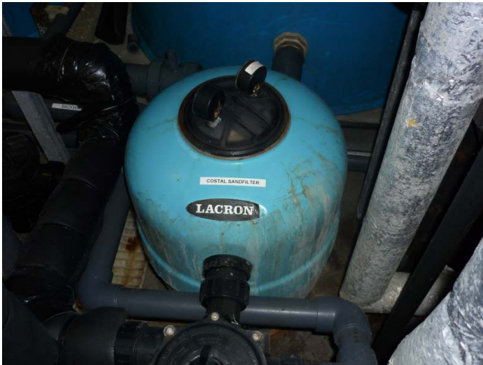
Aquarium Plant room No 1 - Typical sand filter_1.0
