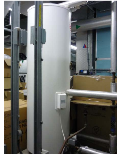
2001 Extension - Kitchen & Toilet HW calorifier_1.0
