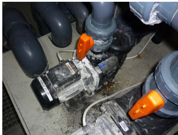
Aquarium Plant room No 9 - Salt contaminated surge pump_1.0
