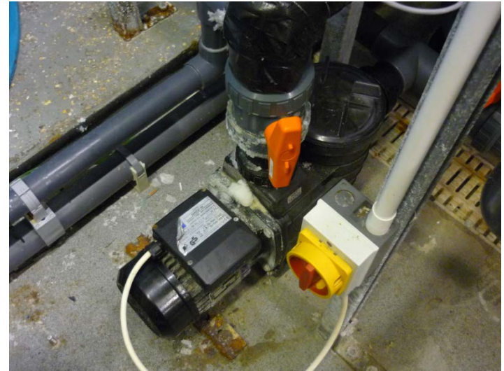
Aquarium Plant room No 1 - Backwash Pump severe salt deposits_1.0
