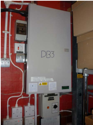
SCC - Typical electrical distribution board_1.0
