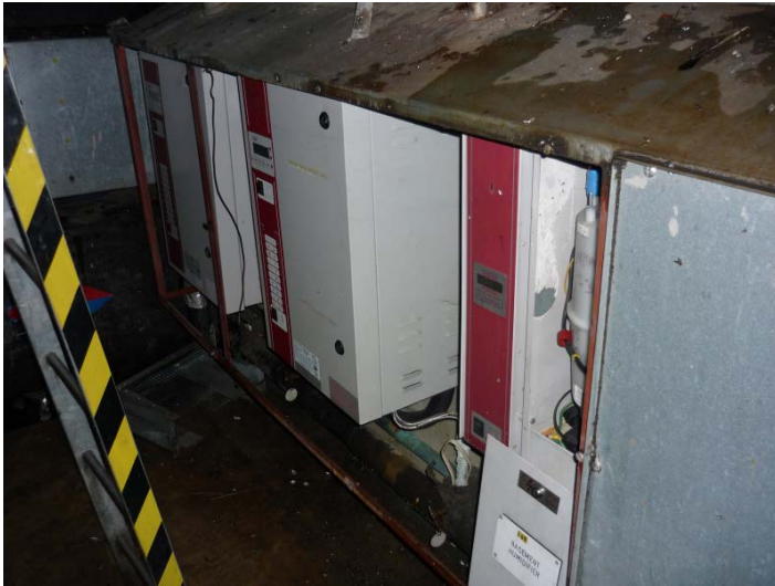
South Hall basement court yard - Dilapidated humidifiers_1.0
