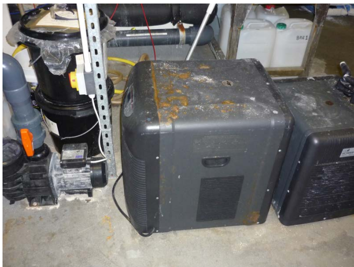
Aquarium Plant room No1 - Temporary AC unit_1.0
