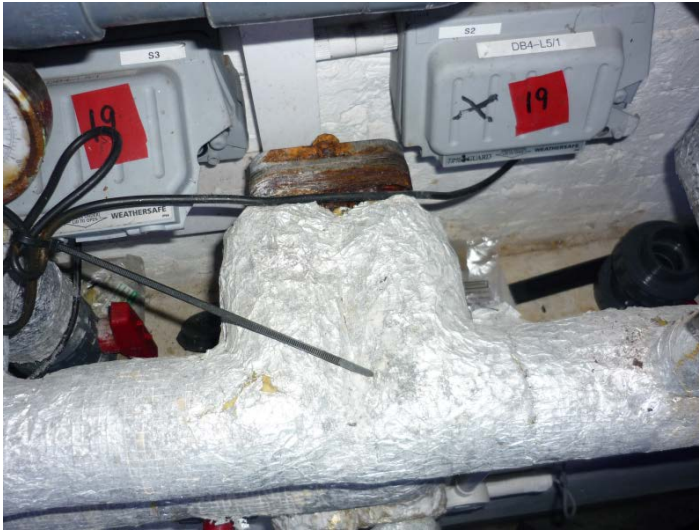
Aquarium Plant Room 4 - Poorly installed plate heat exchanger_1.0
