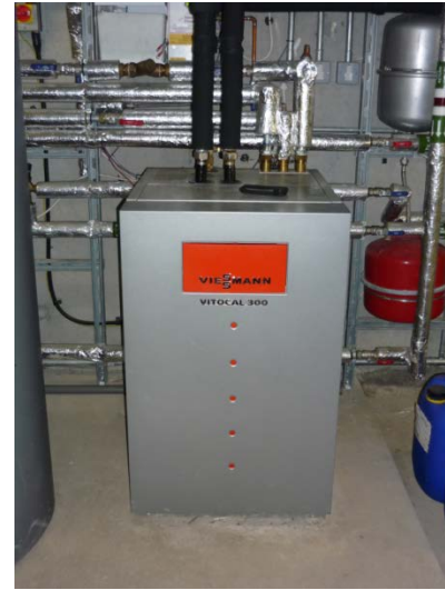
The Pavillion - Ground Source heat pump_1.0
