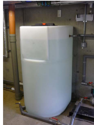
The Pavillion - Cold Water Storage Tank_1.0
