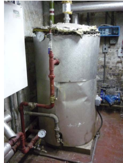
South Hall Boiler room - HW Calorifier_1.0
