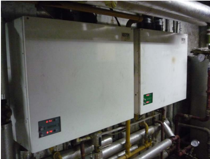
South Hall Boiler Room - Gas fired Boilers_1.0
