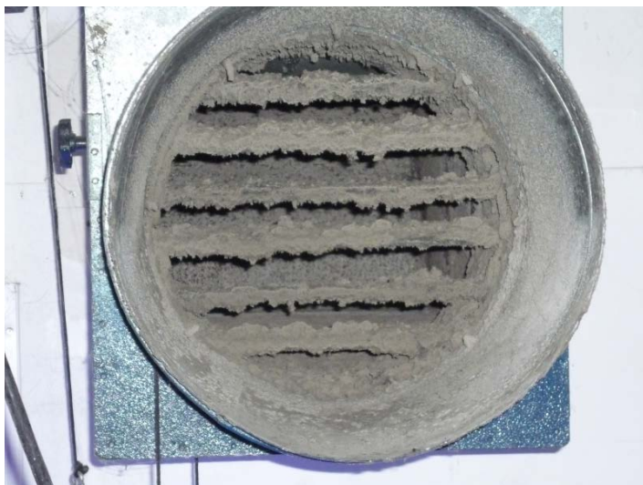
Aquarium Plant Room No 5 - Heavily contaminated ventilation duct_1.0
