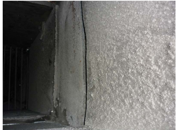
South Hall Boiler room - Contaminated internal ducting_1.0
