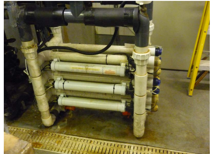
Aquarium Plant Room No 1 - Typical UV lamp array_1.0
