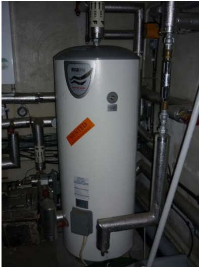
Bothy Building - Ground floor HW Calorifier_1.0
