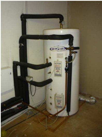
Cue Building - Hot Water Storage heater_1.0
