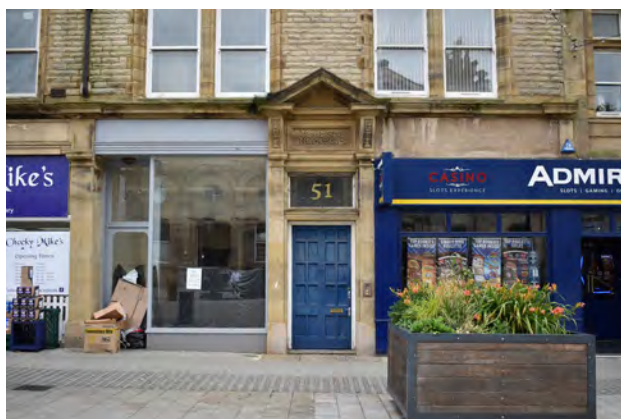
3.1.1.3 Market Chambers (north elevation), original ashlar fascia to bay 1
