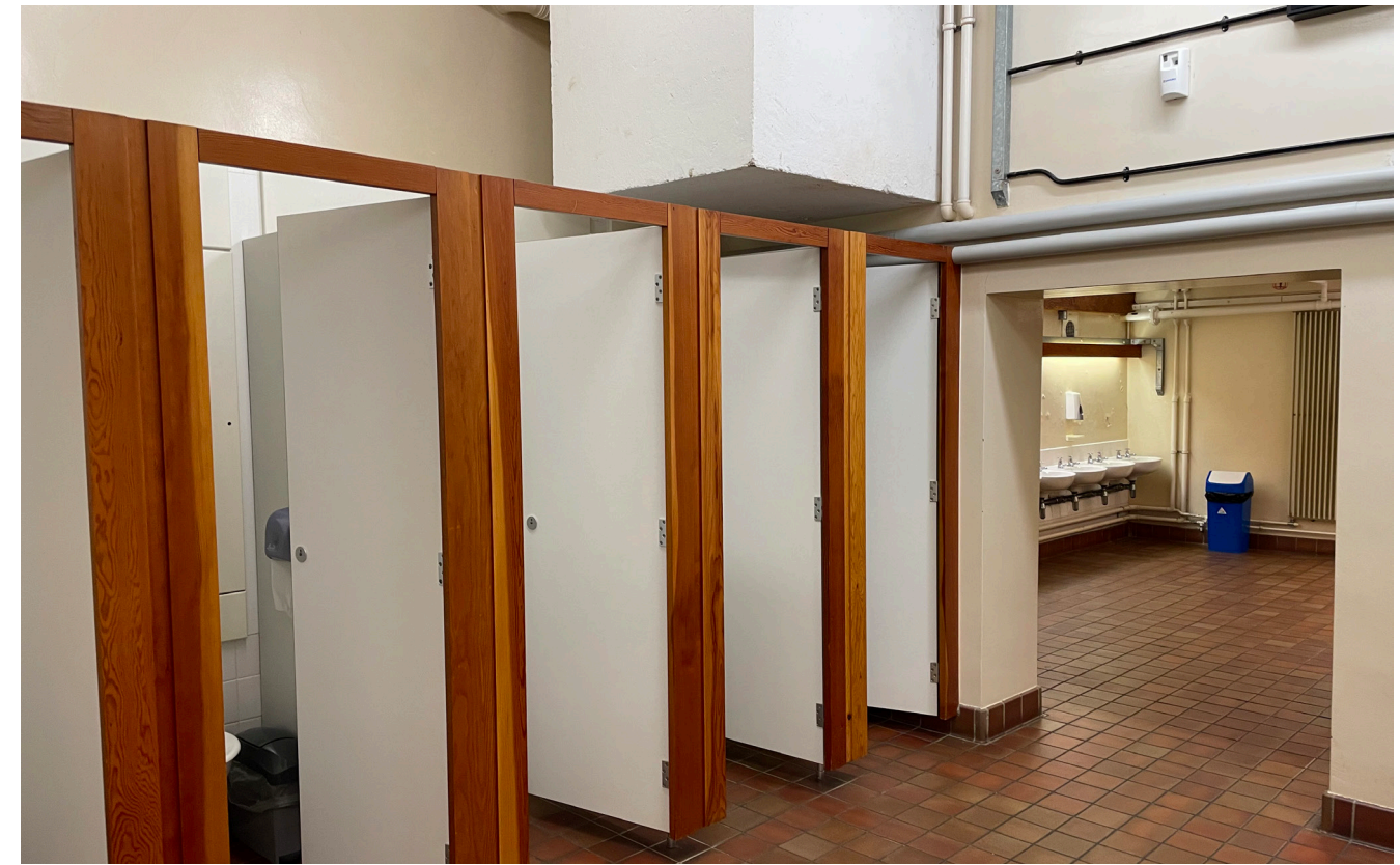
Photograph showing typical WCs as at present
