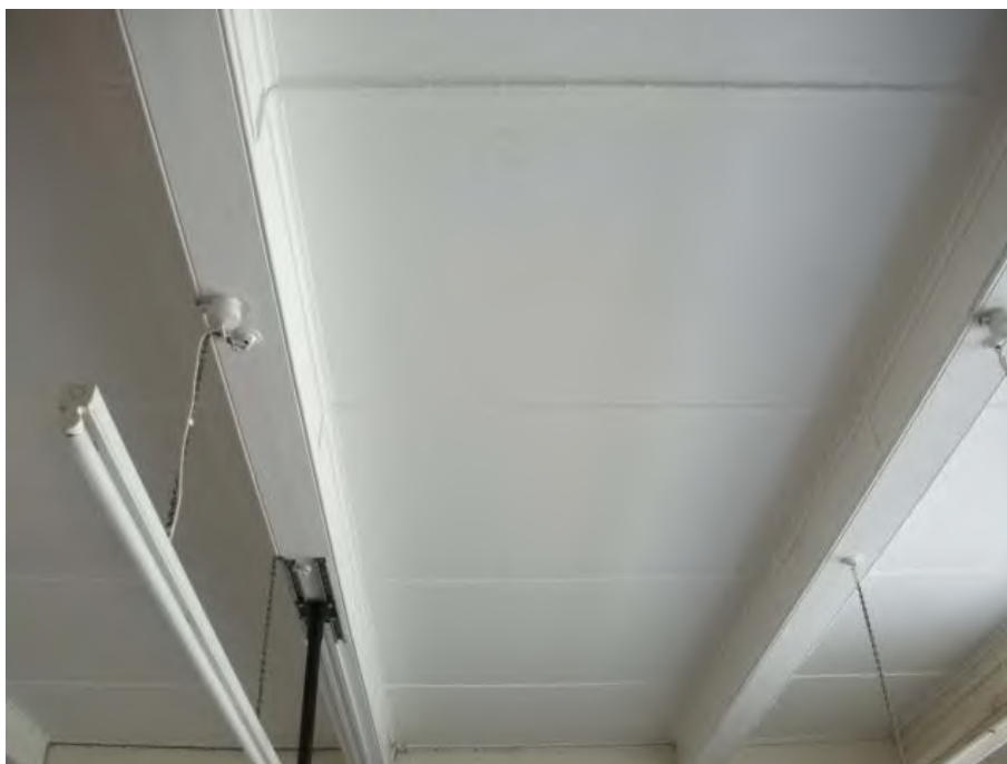
Photo 2: 0/20 Classroom – asbestos cement ceiling
