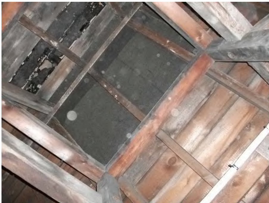
Photo 1: 0/018 Dining/Music – asbestos felt to underside of roof in loft space
