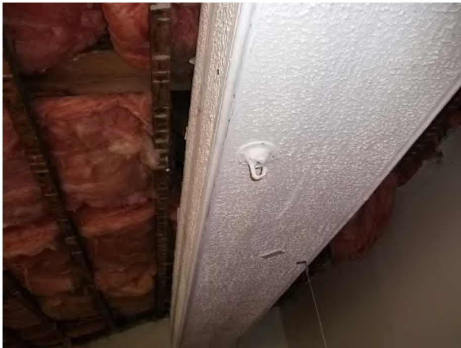
Photo 3: 0/21A Girls WC – Asbestos textured coating in ceiling void
