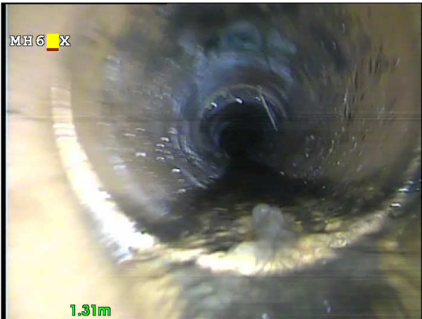
Photo: 43_4a, 00:00:00 1.35m, Joint displaced. Medium
