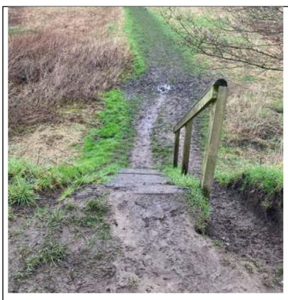
Staircase 4: Remove current timber steps and replace like for like. Steps 1.2m (W) with riser of 20cm – as per Environment Agency Access for all Guidance. Treated timber planks 800 x 200 x 38mm. Infill with 200mm type 1 stone.
