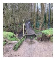
An area of rutting to the embankment. This is required to be dug out, benched and reinstated following the Environment Agency Operational Instruction 110\_07 Technical design details for embankments.
