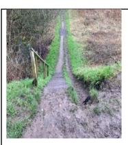
Staircase 2: Remove current timber steps and replace like for like. Steps 1.2m (W) with riser of 20cm – as per Environment Agency Access for all Guidance. Treated timber planks 800 x 200 x 38mm. Infill with 200mm type 1 stone.
