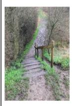
Staircase 3: Remove current timber steps and replace like for like. Steps 1.2m (W) with riser of 20cm – as per Environment Agency Access for all Guidance. Treated timber planks 800 x 200 x 38mm. Infill with 200mm type 1 stone.
