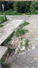
Asset 120567 Staircase replacement and embankment tie-in/repair and rutting.
