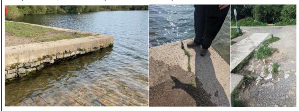
Asset 120567 Staircase replacement and embankment tie-in/repair and rutting.
