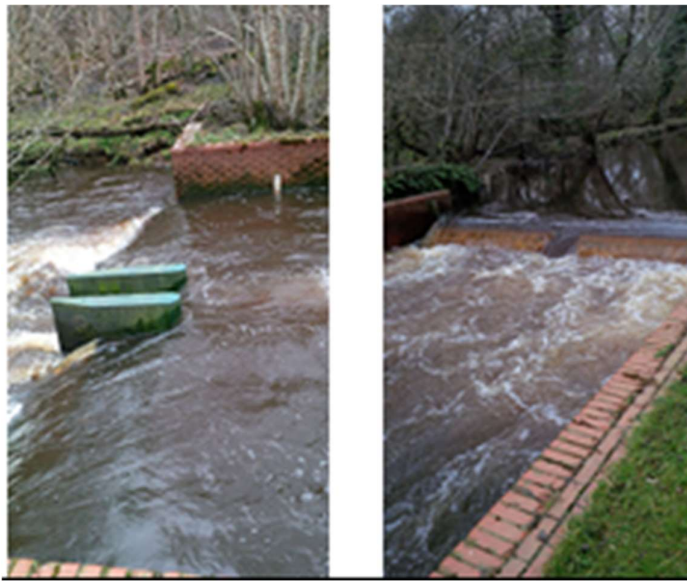
Photo showing the downstream broad crested weir (left) and thin plate gauging weir (right).
