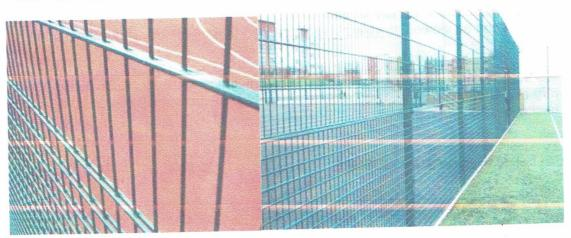
This unobtrusive ball court fence is built to last, as you will see from the pictures, we increase the strength of the lower 1200mm sections to accommodate the stress these areas experience, this is because 90% of all ball impacts are to the lower section, goal backs also have stronger materials used for the same reason.
