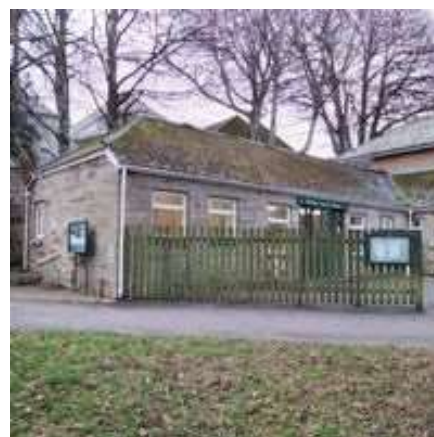
Photo 1. Asbestos Cement Roof Tiles
