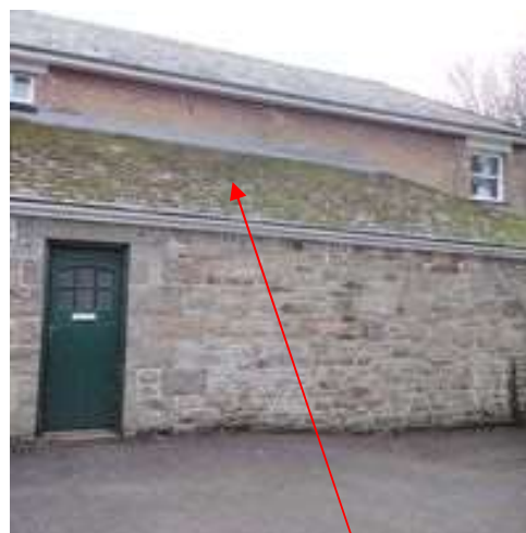
Photo 2. Asbestos Cement Roof Tiles
