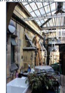
Figure 32: The Flower Store, note metal window on left hand side.
