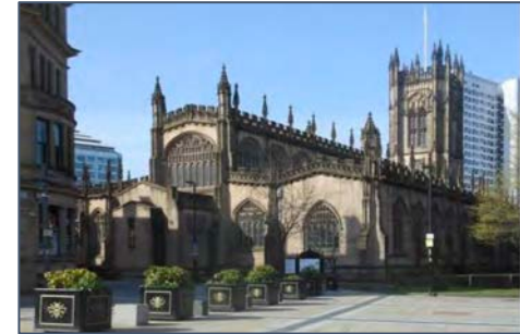
Figure 2: The Cathedral from the east, showing the medieval Choir with lady Chapel and Regimental Chapel (substantially rebuilt post war).
