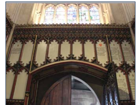
Figure 24: Ground floor of the Tower showing west wall.
