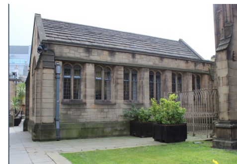
Figure 4: The South-East Annexe (1934).
