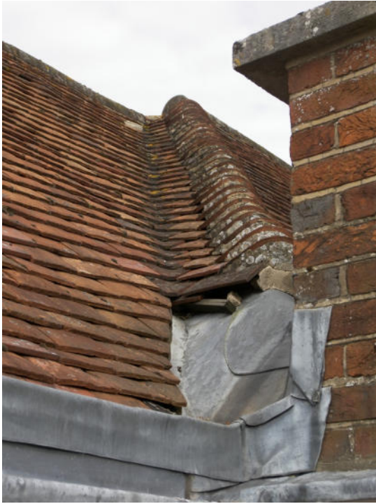
parapet gutter and other details
