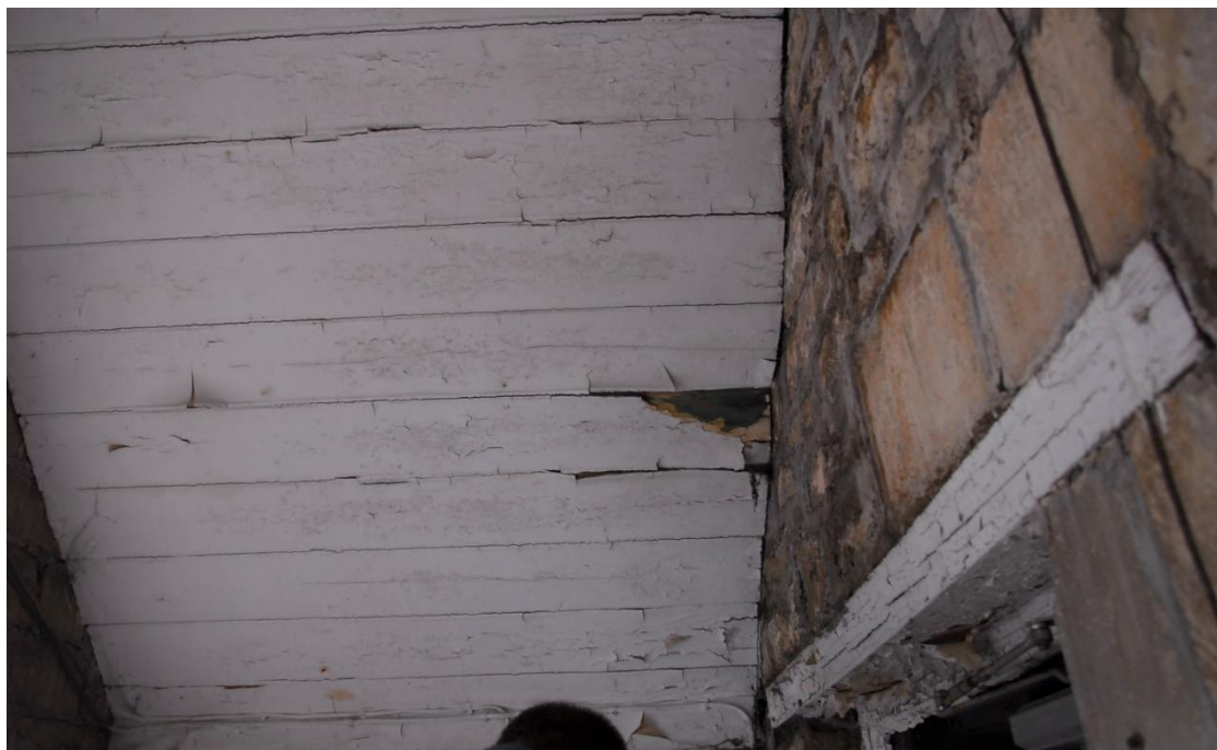
Figure 46 Entrance porch ceiling
