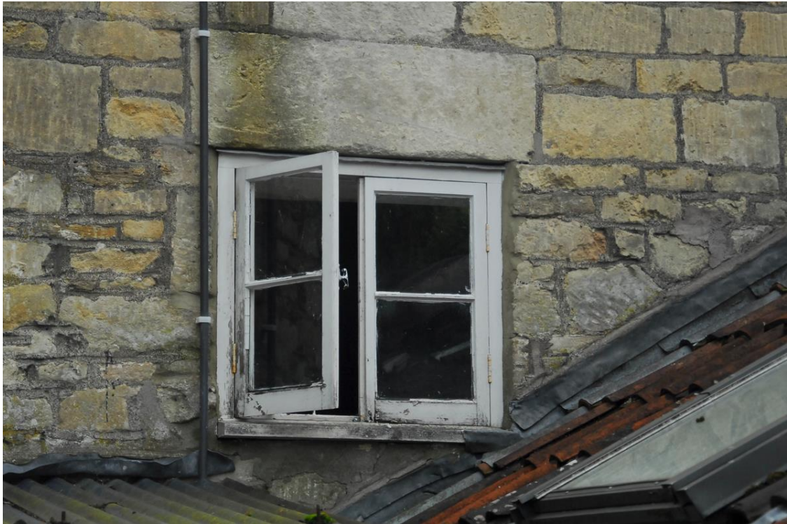
Figure 42 WF5 Timber casement windows
