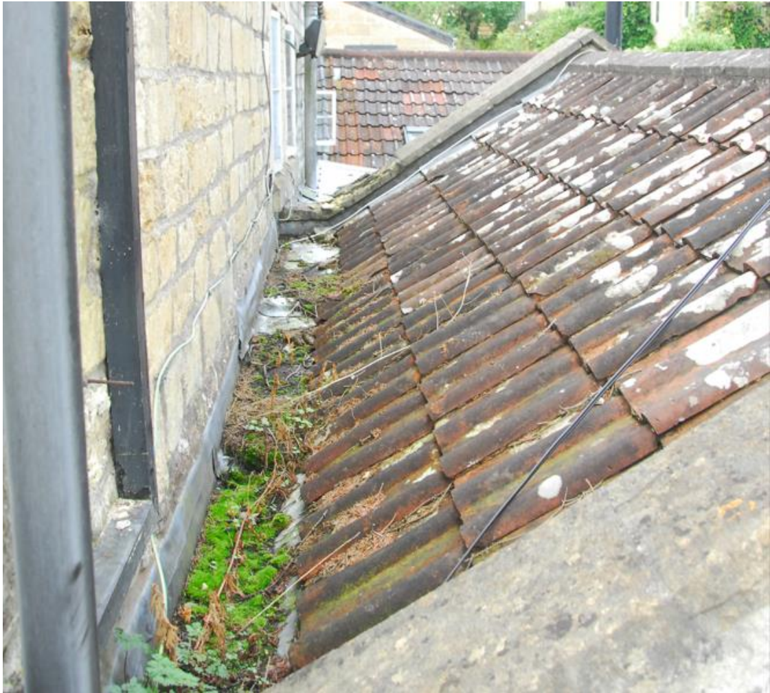
Figure 14 RS 8 Valley Gutter
