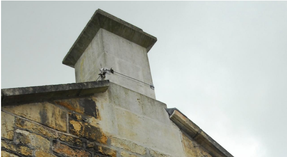
Figure 1 West elevation of CH1
