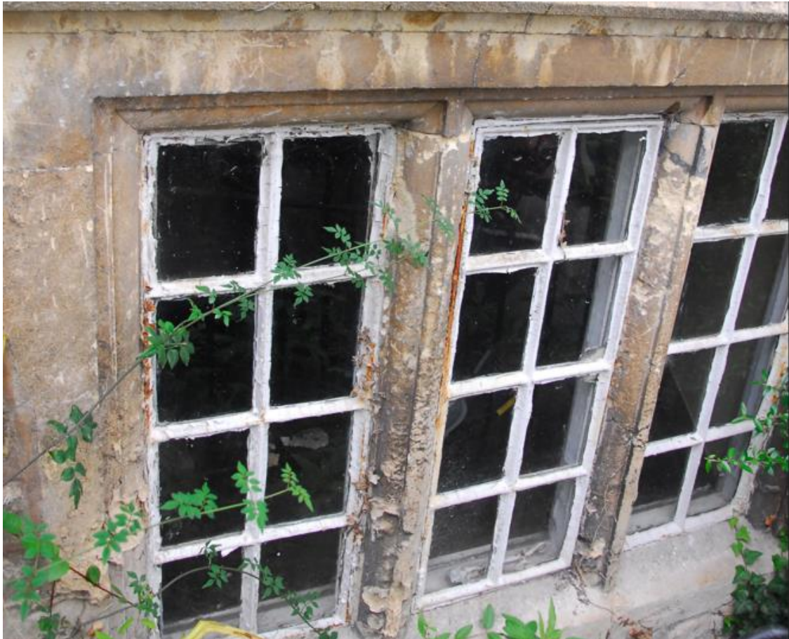
Figure 34 WG1 Metal casement windows
