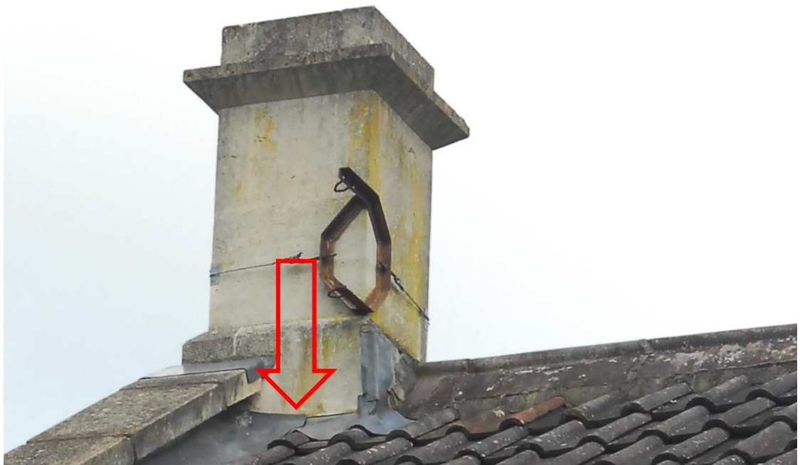
Figure 2 East elevation of CH1
