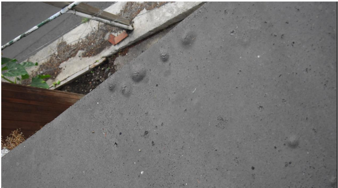
Figure 11 Blistering to RS 6
