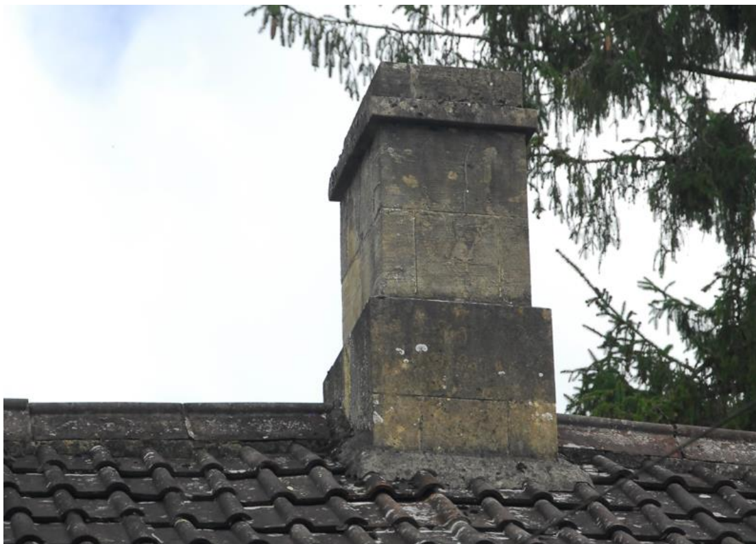
Figure 3 South elevation of CH2
