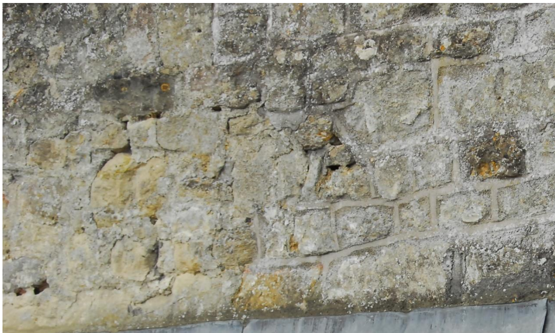
Figure 24 Typical open joints in stonework
