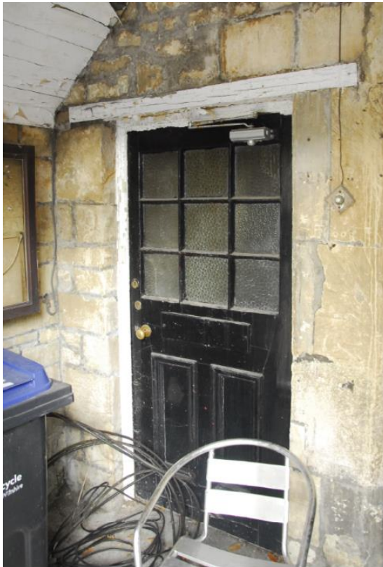
Figure 26 DG1 inserted door
