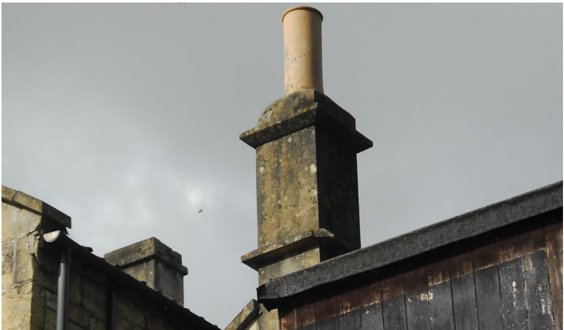
Figure 5 East elevation of CH4
