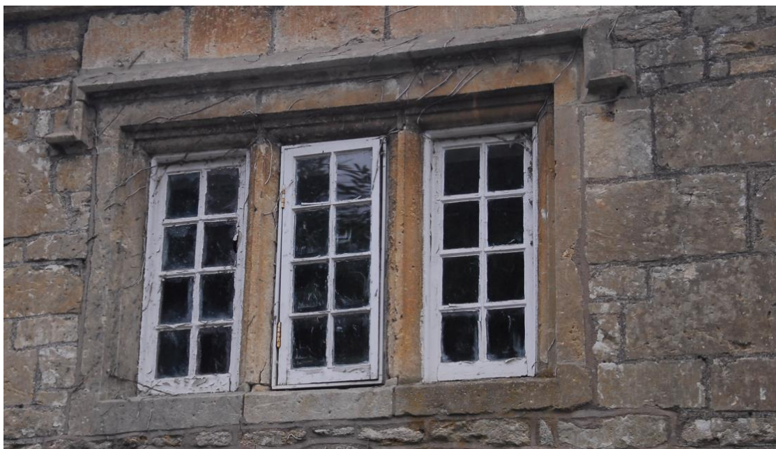
Figure 38 WF1 Timber casement windows
