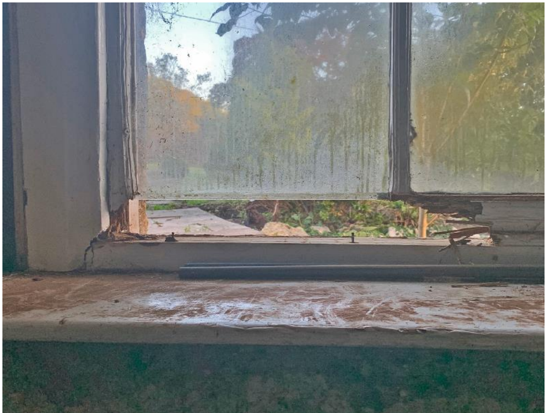
Figure 37 WG4 Metal casement windows
