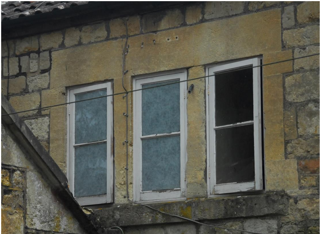
Figure 41 WF4 Timber casement windows
