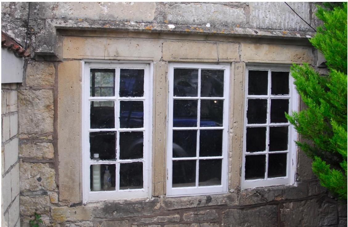
Figure 36 WG3 Timber casement windows
