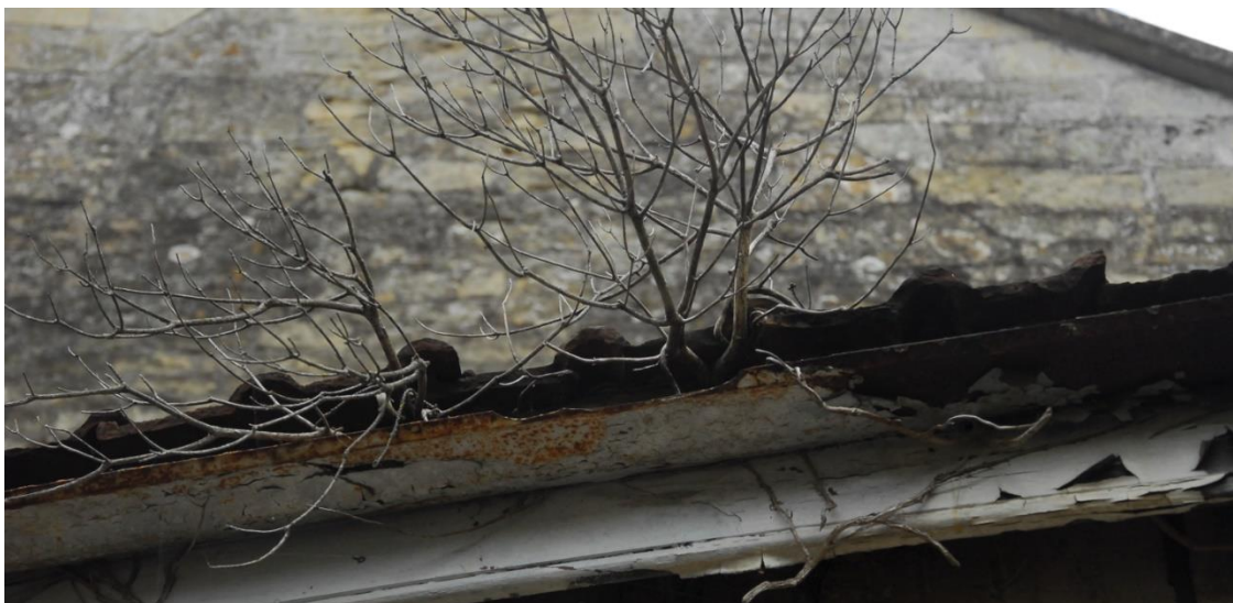
Figure 21 Gutter to RS5
