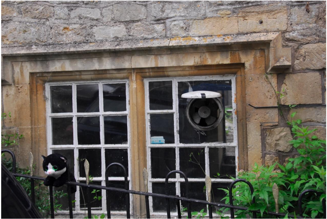
Figure 35 WG2 Metal casement windows
