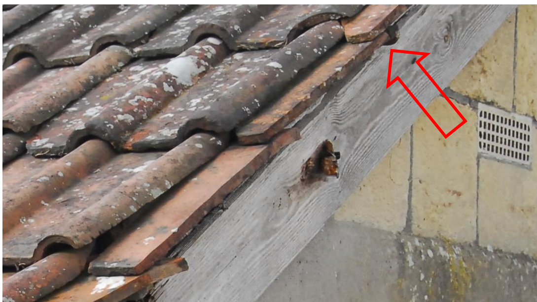
Figure 20 Minimal headlap and open flutes
