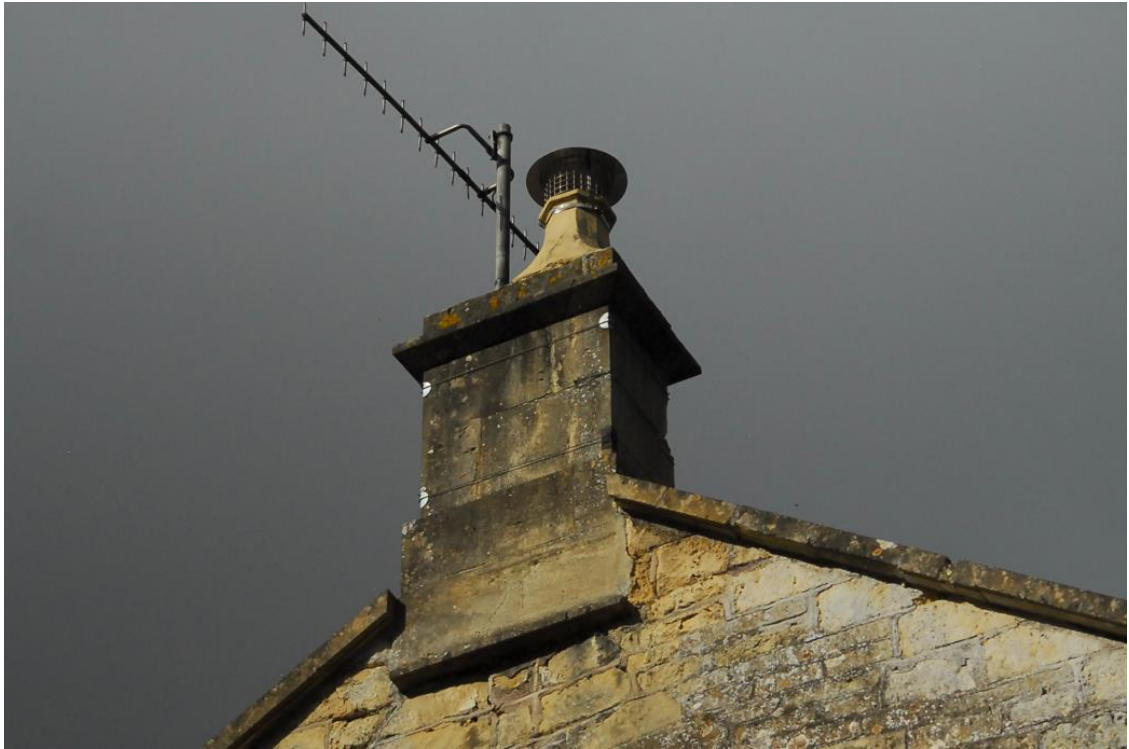
Figure 4 East elevation of CH3
