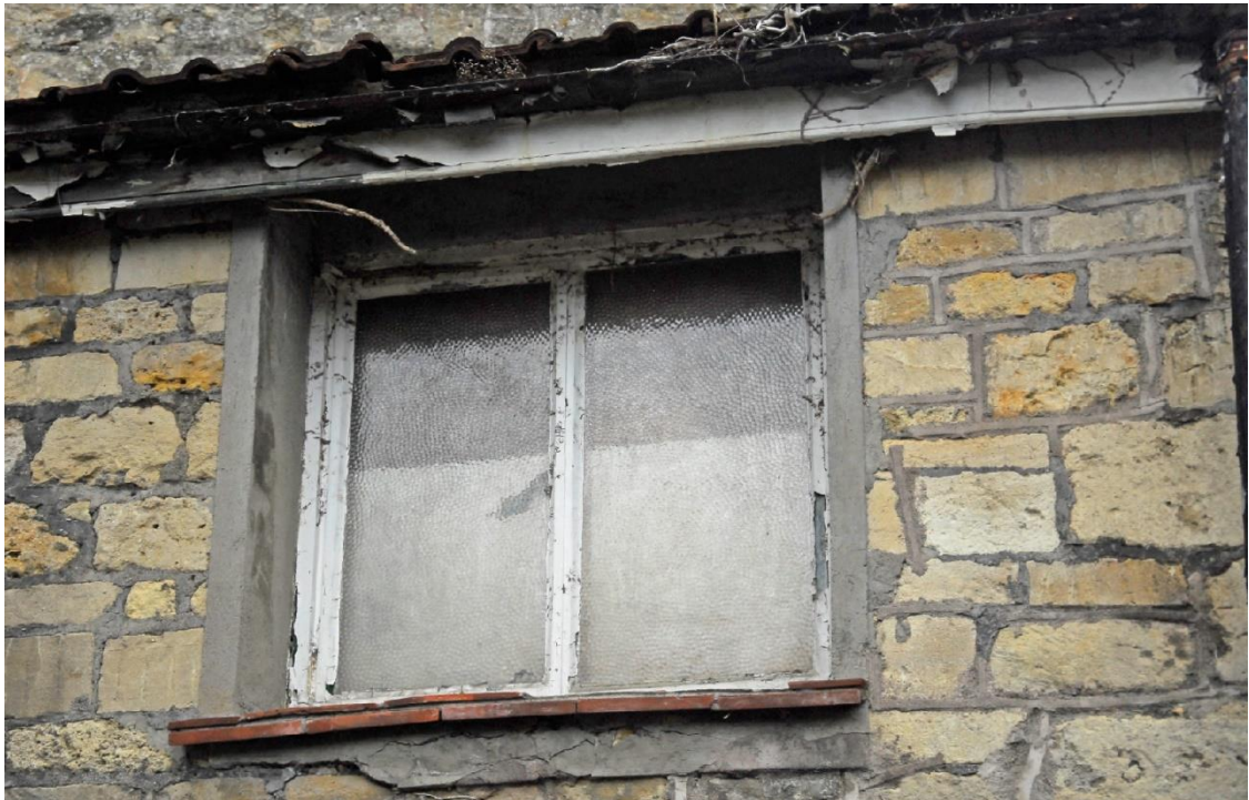
Figure 37 WG4 Metal casement windows
