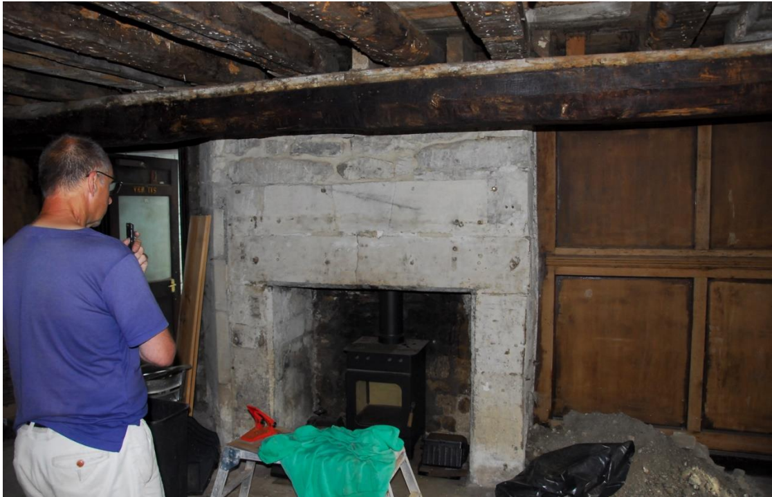
Figure 44 G3 Exposed ceiling structure
