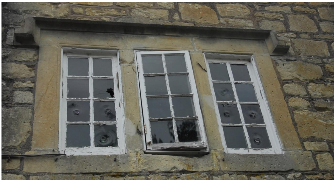
Figure 40 WF3 Timber casement windows
