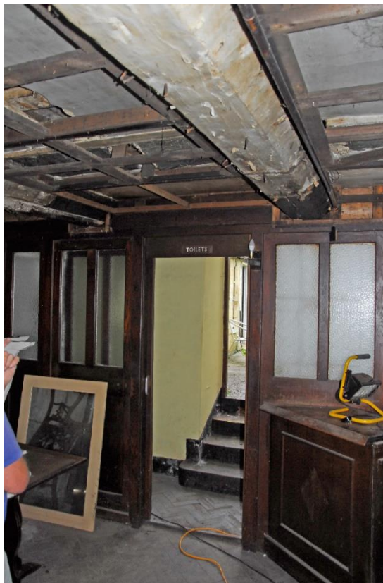
Figure 32 DG16 1960's glazed partition
