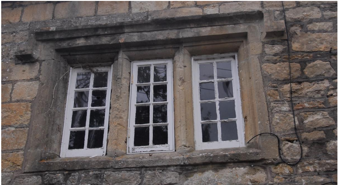
Figure 39 WF2 Timber casement windows
