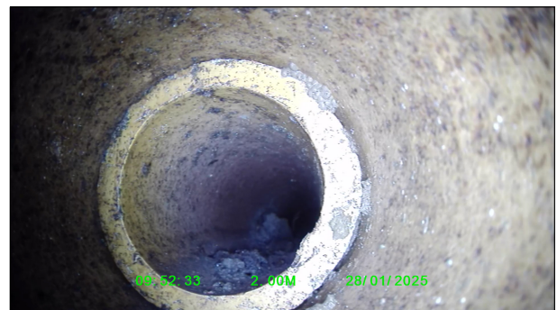
Photo: 4_4_46_A.jpg 2.1m, Shape changes to circular, 75mm high
