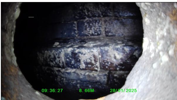
Photo: 3_3_36_A.jpg 8.6m, Finish node type, manhole reference number: Main Sewer Remarks: suspected Main Sewer in Carpark
