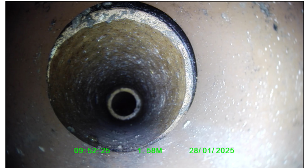
Photo: 4_4_43_A.jpg 1.7m, Material changes, vitrified clay
