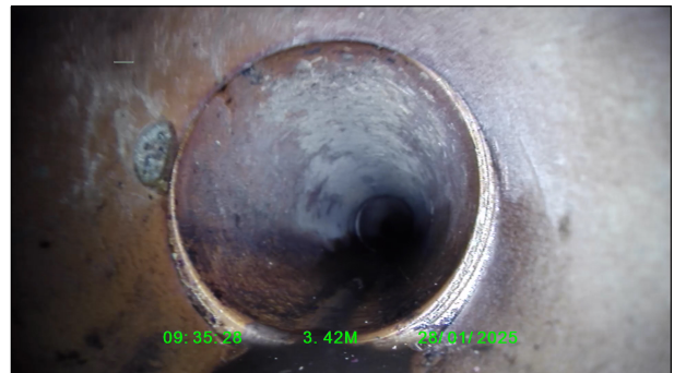
Photo: 3_3_30_A.jpg 3.4m, Line deviates right Remarks: 15deg approx
