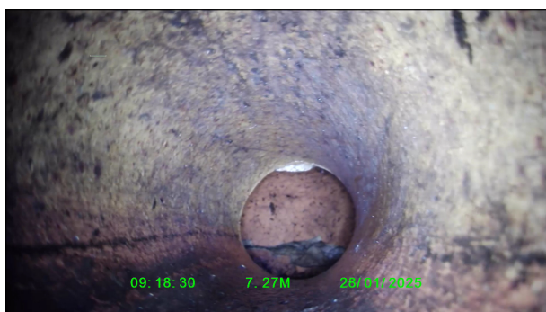
Photo: 1_1_20_A.jpg 7.3m, Line deviates right Remarks: 15deg approx
