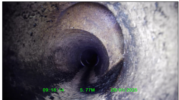
Photo: 1_1_16_A.jpg 5.8m, Junction, at 2 o'clock, diameter 100mm Remarks: unconfirmed source
