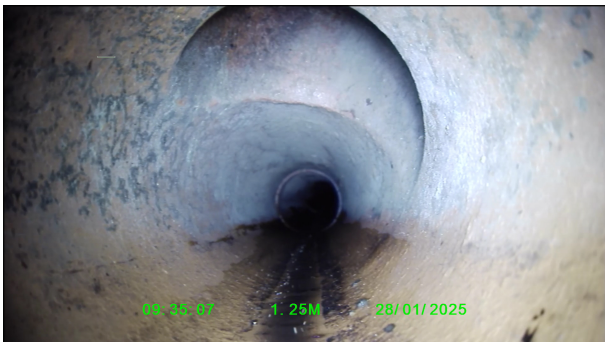
Photo: 3_3_29_A.jpg 1.3m, Junction, at 1 o'clock, diameter 100mm Remarks: unconfirmed source
