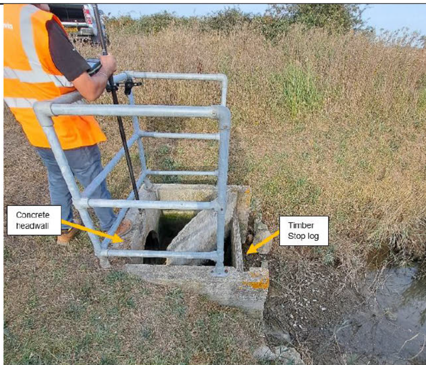
Figure 3- Inlet Structure.
