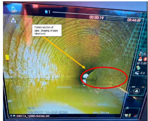
Figure 8- CCTV image (01/2024) taken from penstock chamber towards inlet.
