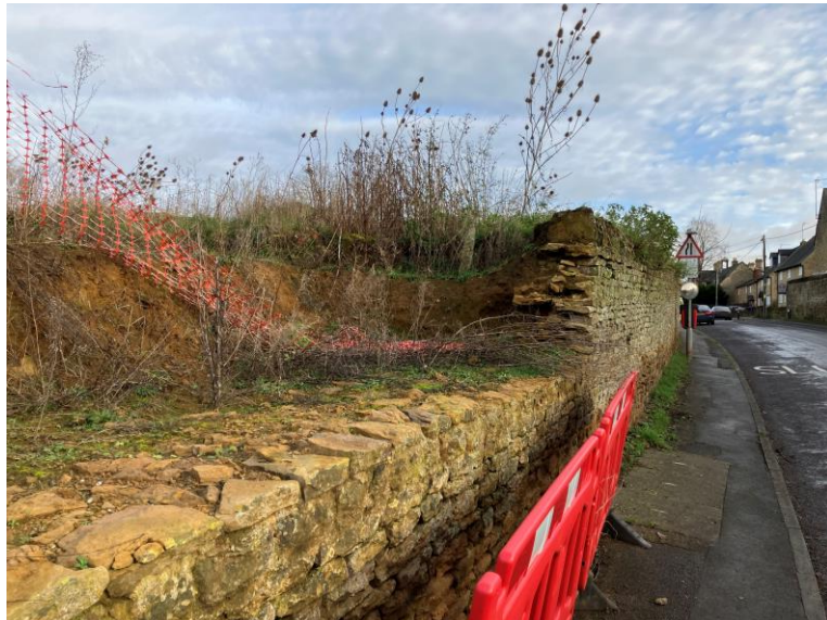
Three pictures showing cross section of the current wall and the 2 areas where existing wall has been removed following collapse
