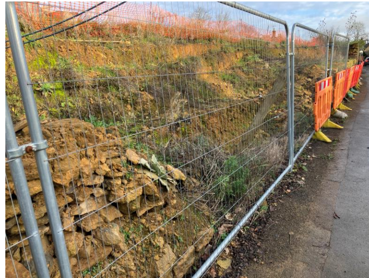
Three pictures showing cross section of the current wall and the 2 areas where existing wall has been removed following collapse
