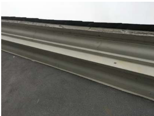
Photograph 11. Tightly fitted soffit of R3.
