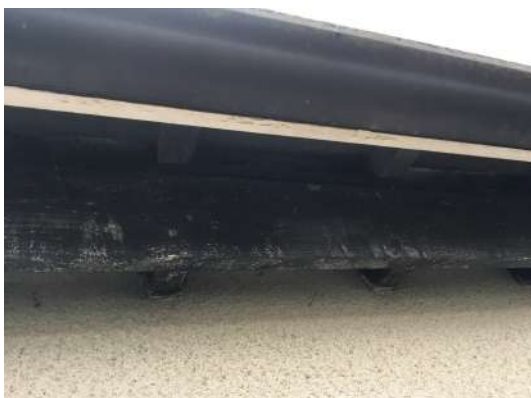
Photograph 13. Gaps between the rafters at the eaves of R4.
