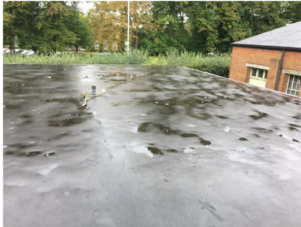
Overview image of roof shows falls are minimal so some standing water does occur
