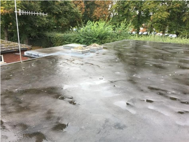
Overview of roof area
