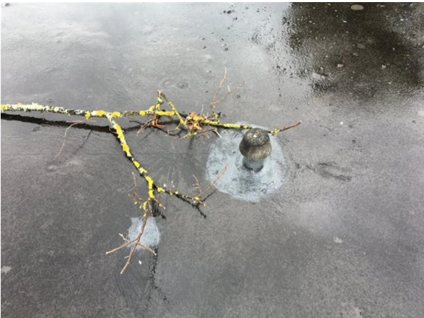
Screed vent to be removed
