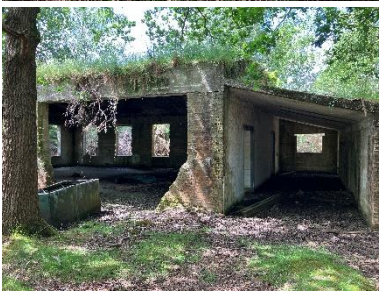
Windows (south). Openings (south)
