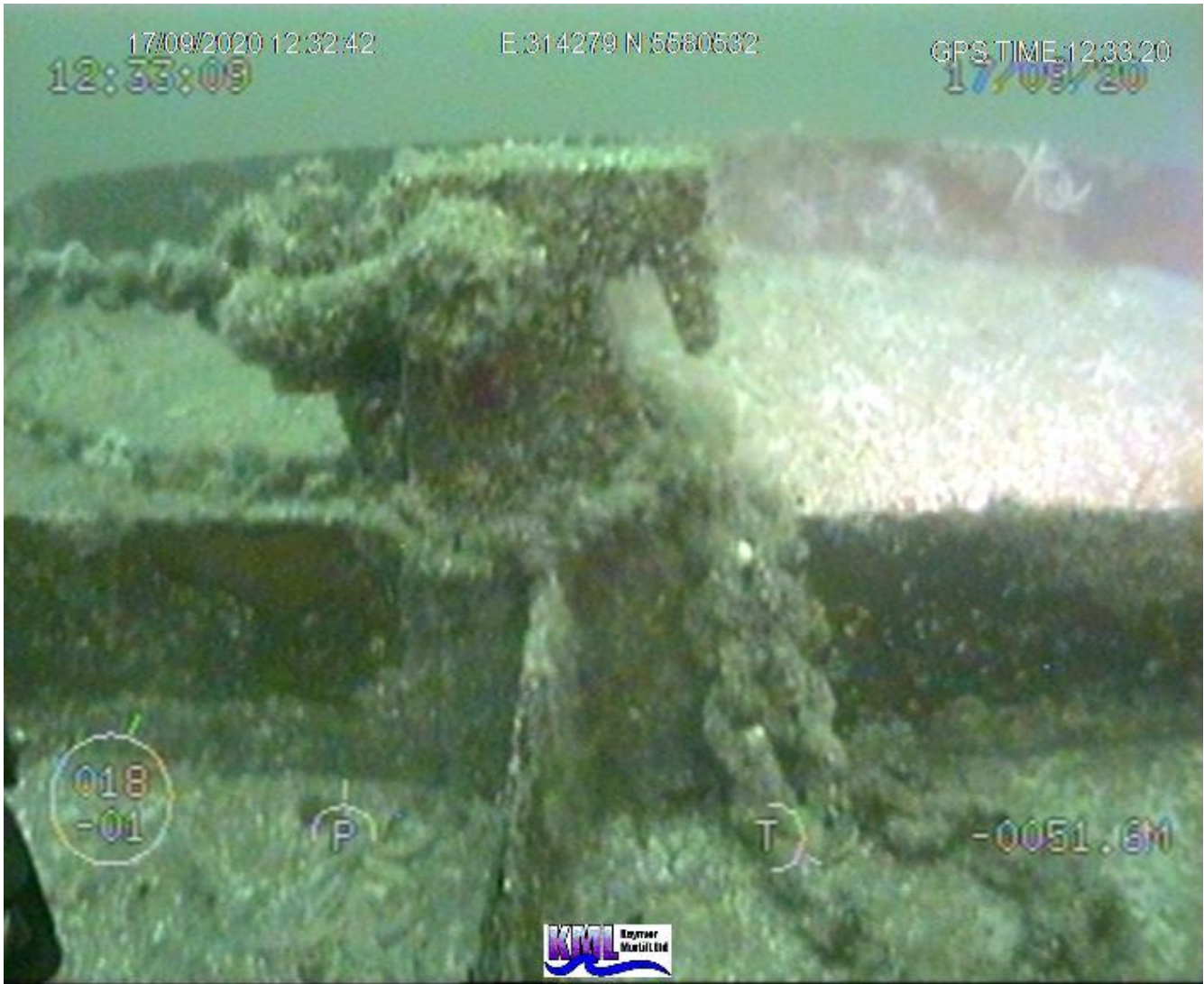
(vii) NE mooring clump top connection opposite angle
