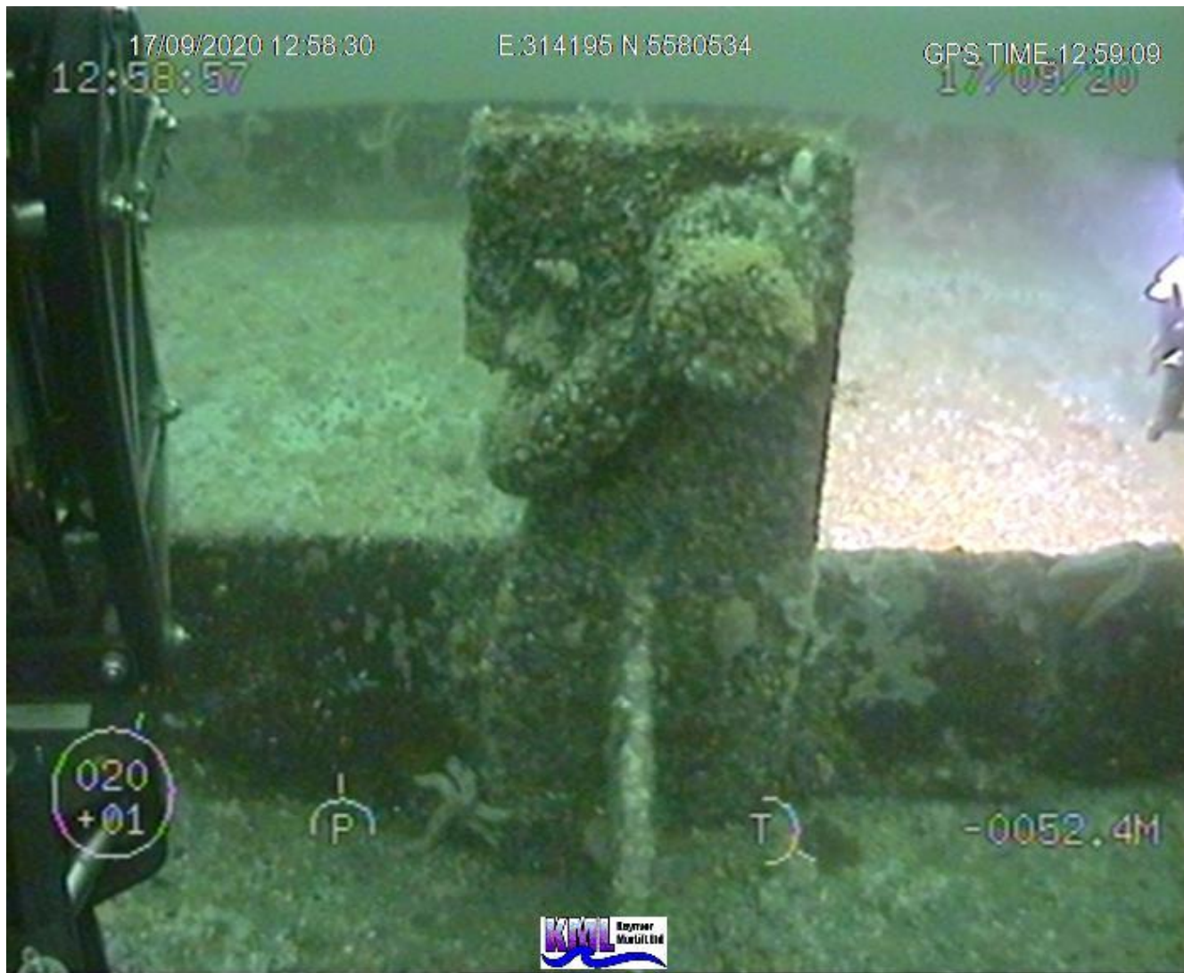
(ix) NW mooring clump top connection
