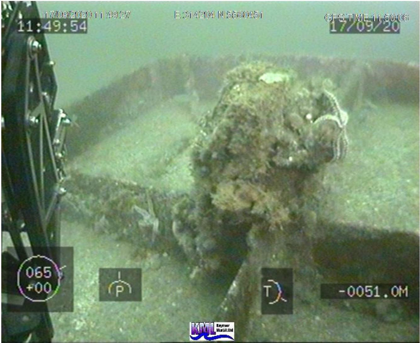
(iv) SW mooring clump top conenction
