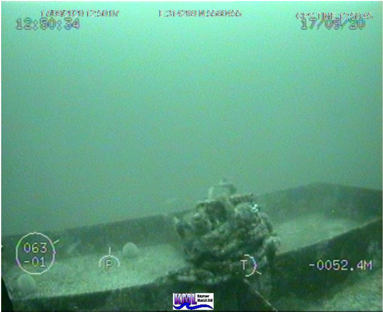
(iii) SE mooring clump top connection. Some dyneema remaining.
