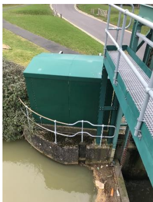
Photo 6 – High level walkway
