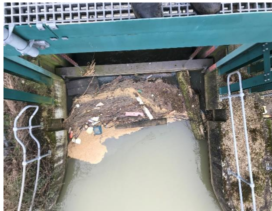
Photo 5 – Middle sluice light position
