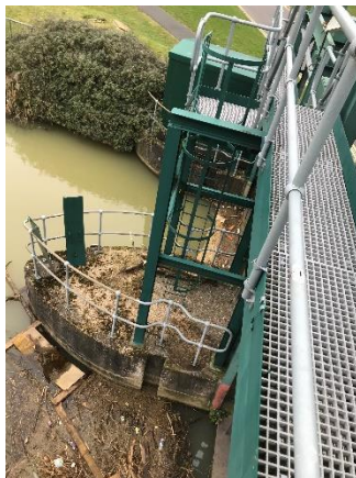
Photo 4 – Vertical access ladder
