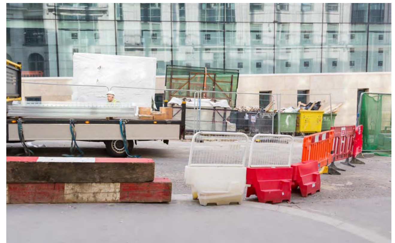
Bad practice: multitude of mixed barrier types, which are not assembled into a continuous barrier
