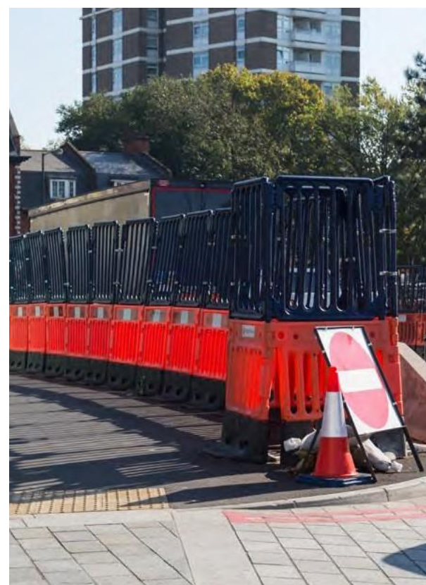
Straight and tidy barriers maximise safety and give a good impression on site
